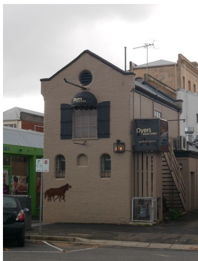
Figure 31. (left) Former Titheridge and Growcott real estate office, 15-19 Main Road [HO93] (GJM Heritage, November 2021).
