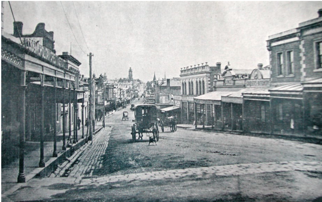
Figure 6. Looking west down Bridge Street from Bakery Hill. On the right are the buildings currently occupied by McDonald's restaurant. Note bluestone kerbs with verandah posts fixed to them and wide bluestone channels along the street [photo undated, prior to Bridge Street tramline installed post-1904] (Source: Victorian Collections, ID 3323).
