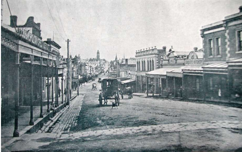
Figure 6. Looking west down Bridge Street from Bakery Hill. On the right are the buildings currently occupied by McDonald's restaurant. Note bluestone kerbs with verandah posts fixed to them and wide bluestone channels along the street [photo undated, prior to Bridge Street tramline installed post-1904] (Source: Victorian Collections, ID 3323).
