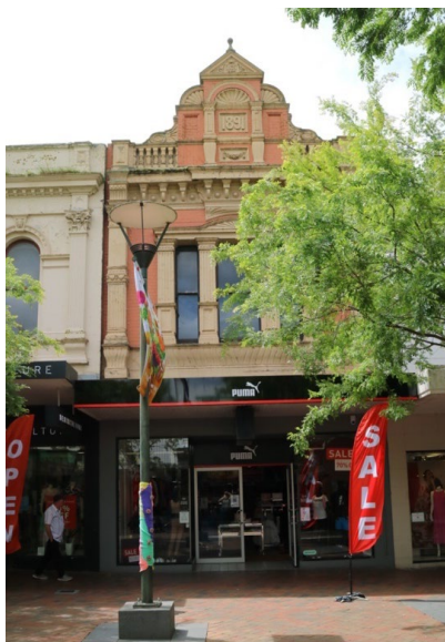
Figure 26. (left) 24-26 Bridge Mall (GJM Heritage, November 2021).
