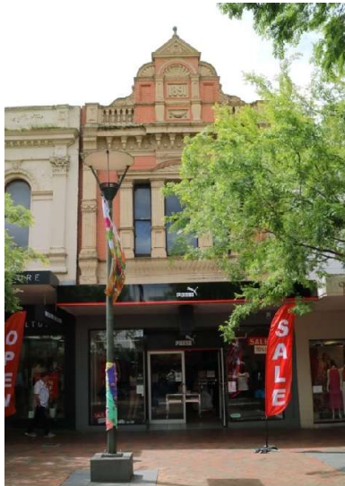
Figure 26. (left) 24-26 Bridge Mall (GJM Heritage, November 2021).
