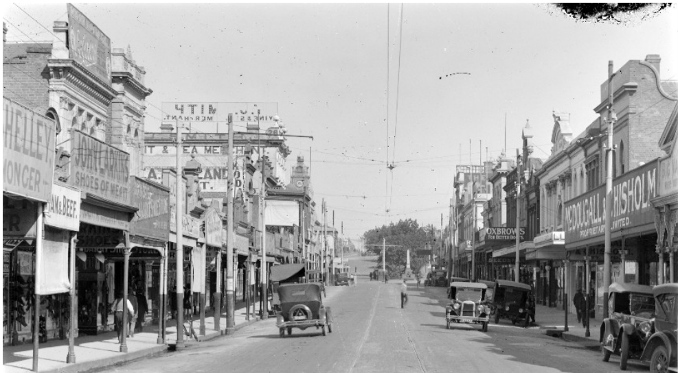
Figure 7. Looking west down Bridge Street, c1920s/30s (SLV, Rose Series P3165, ID 1768215).
