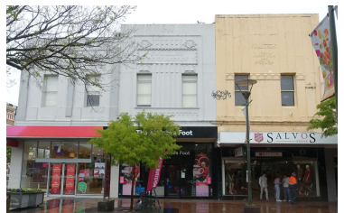
Figure 20. (left) No. 90 Bridge Mall, showing Peel Street elevation (Landmark Heritage, October 2022).
