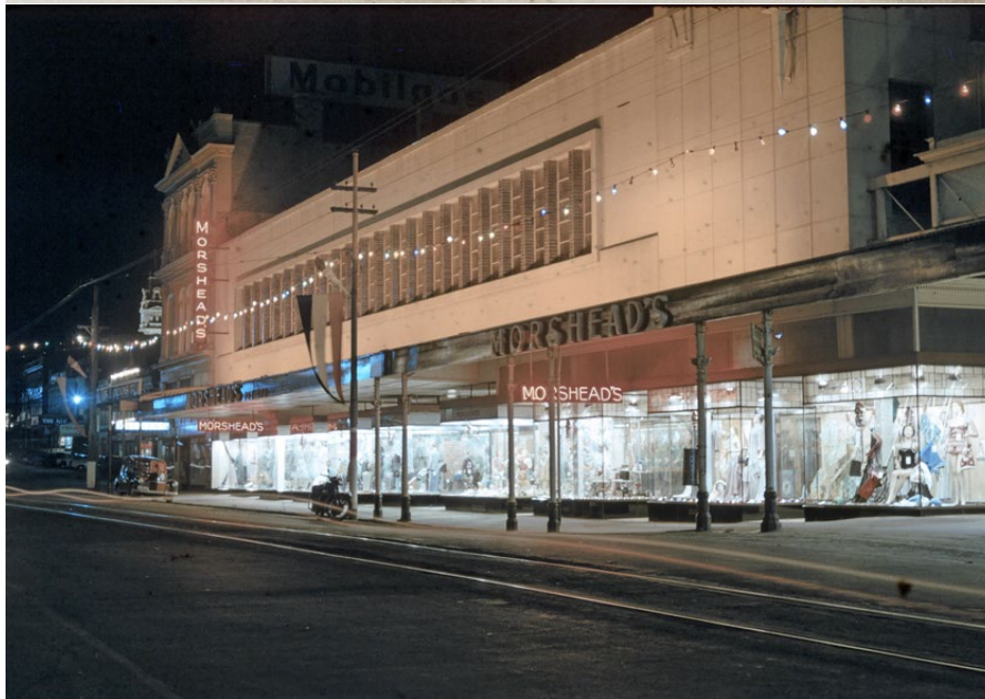
Figure 11. Morshead's Department Store showing the c.1952 façade and their famous illuminated window displays (Source: Victorian Collections https://victoriancollections.net.au/items/595f2b9ed0cdd325c0a4e53c , accessed 7 July 2024). Looking east up Bridge Street, from Sturt Street, 1938. Left is the Victorian building occupied by Bean Son & Co., altered c.1960s (as Morshead's Department Store) and c.1980s to form Norwich Plaza (Source: Ballarat Revealed).
