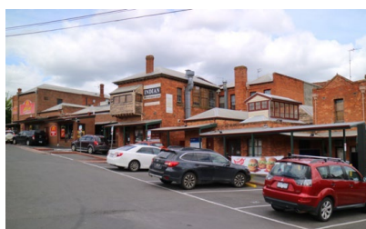
Figure 18. (left) Nos. 44-22 Main Road (left to right) (GJM Heritage, November 2021).
