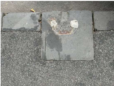
Figure 23. (right) Large kerb block with remnant marks where a verandah post was fixed (City of Ballarat, January 2023).
