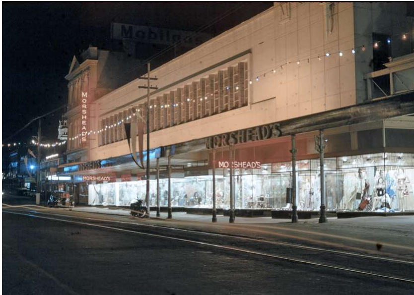
Figure 11. Morshead's Department Store showing the c.1952 façade and their famous illuminated window displays (Source: Victorian Collections https://victoriancollections.net.au/items/595f2b9ed0cdd325c0a4e53c , accessed 7 July 2024).
