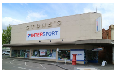
Figure 16. (left) Intersection of Bridge Mall, Grenville Street and Sturt Street. Norwich Plaza to the centre left of image (GJM Heritage, June 2021).
