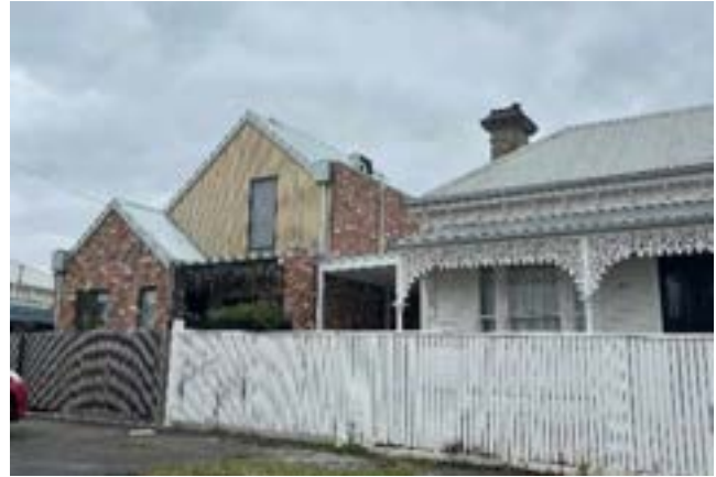
Infill development in Ballarat East Photo by Ethos Urban
