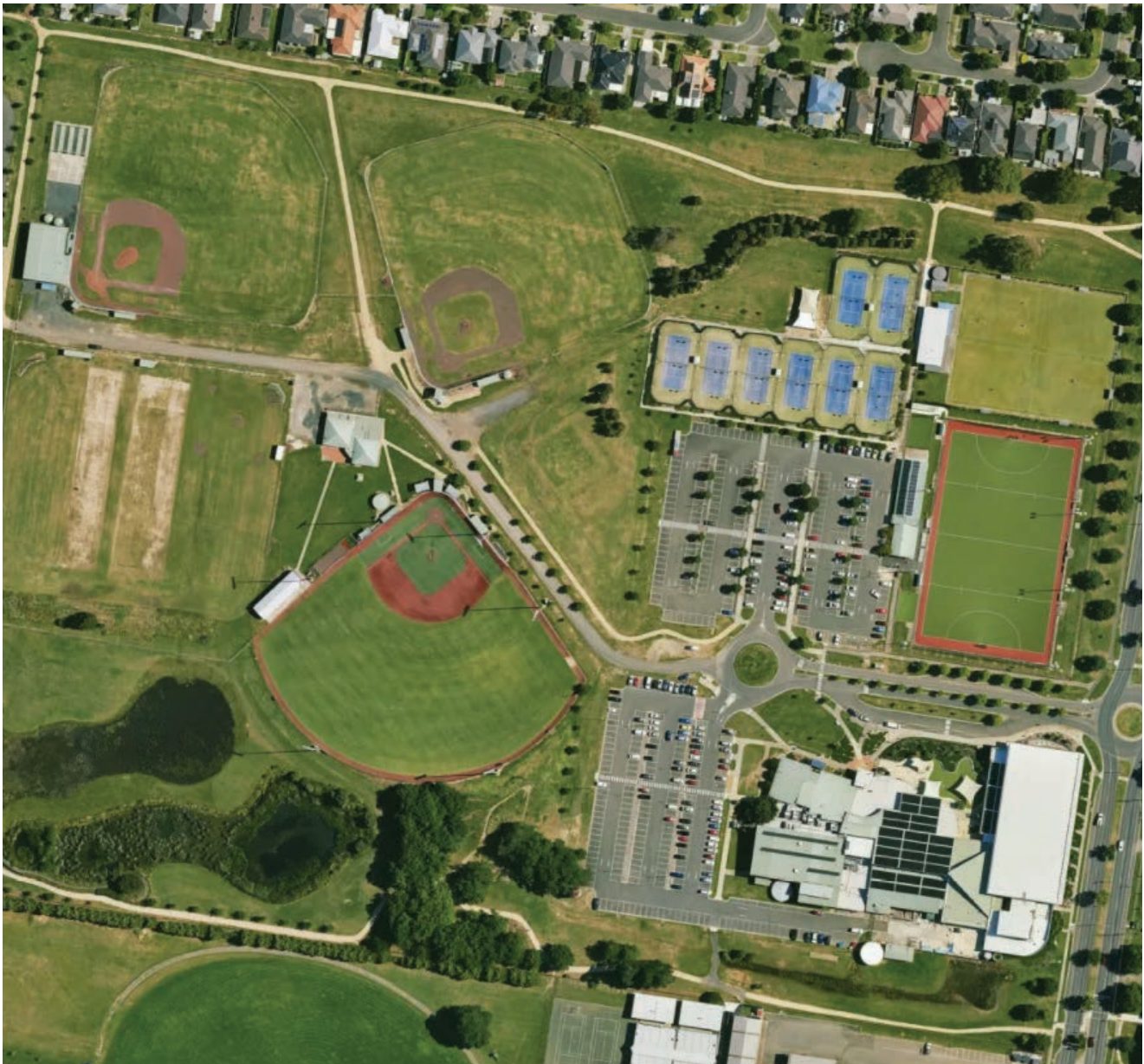
Figure 1: POWP Aerial View - Site Layout
