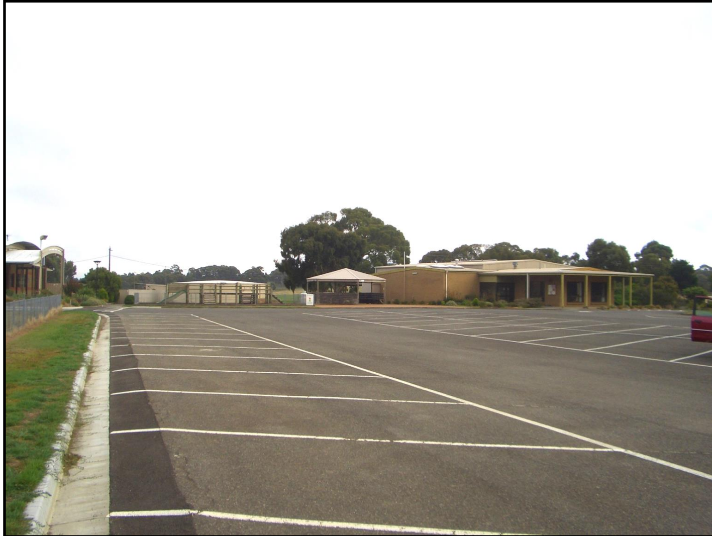
(i) Car parking area and major buildings at the Invermay Recreation Reserve.
