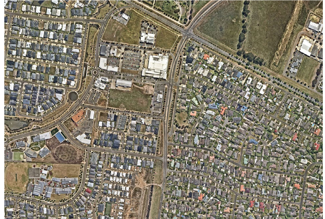
Site Aerial as of 7 November 2023
