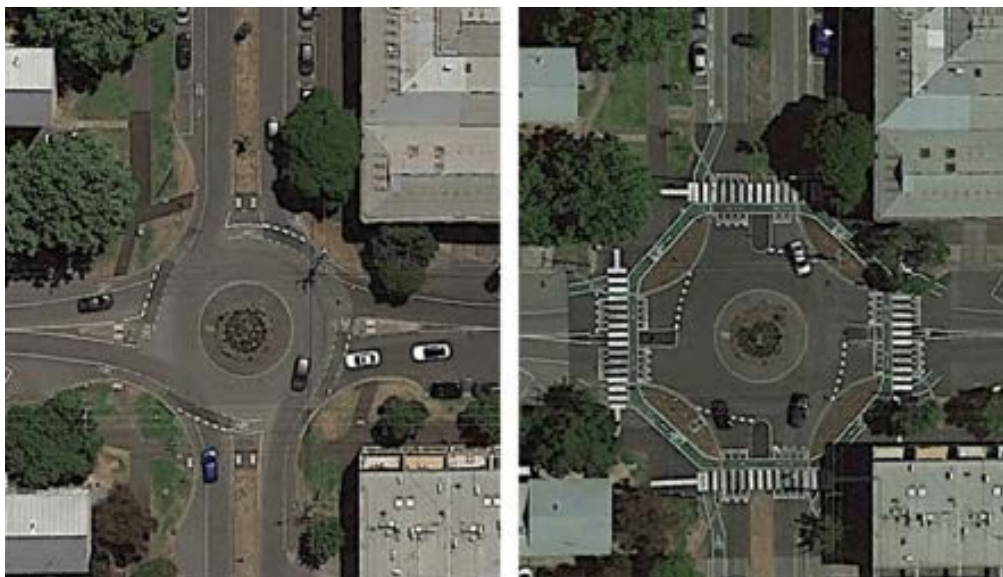
Figure 14 -before and after the treatment is applied in Figure 13 at Moray St, South Melbourne
