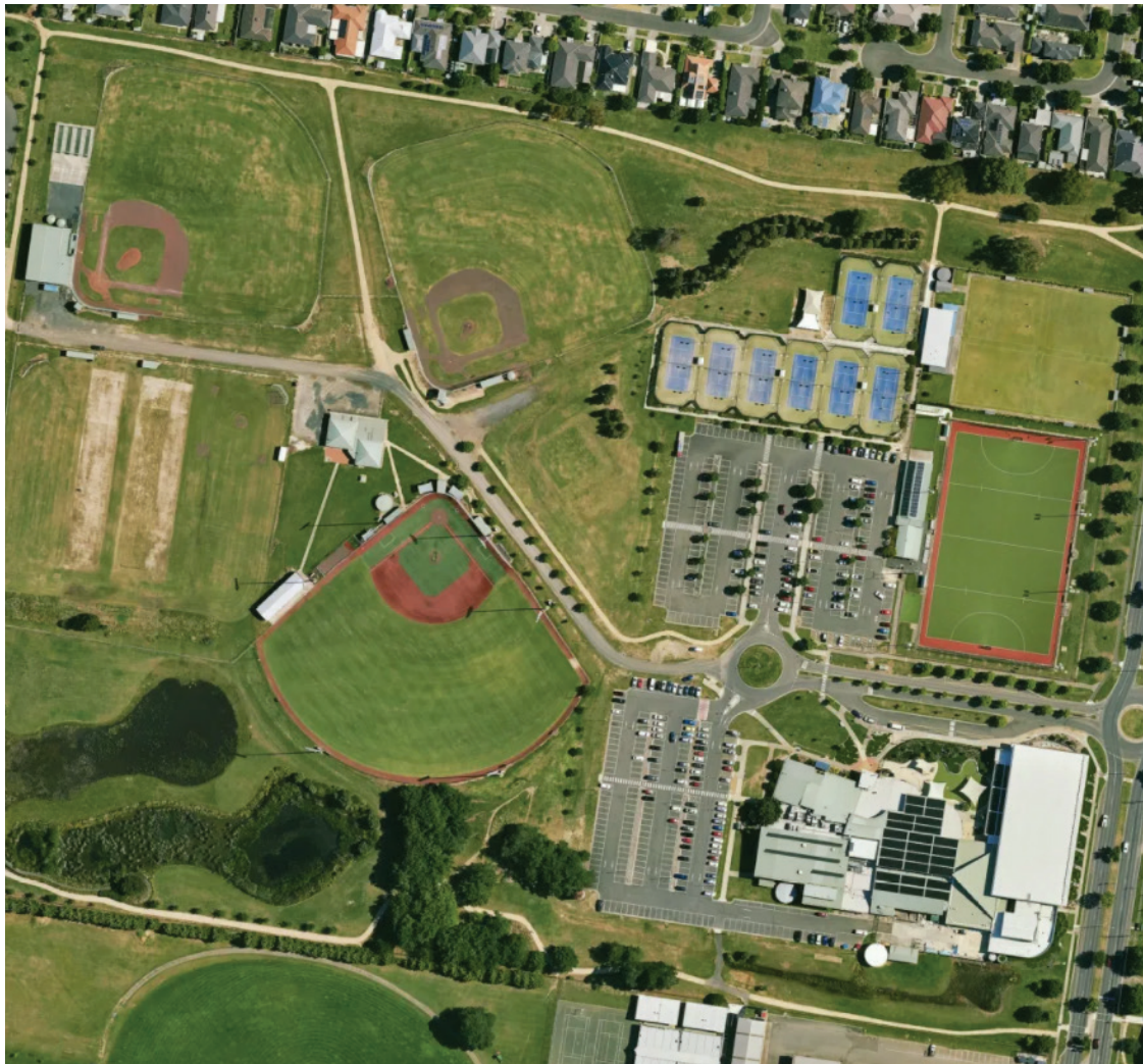
Figure 1: POWP Aerial View - Site Layout
