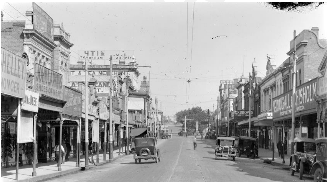
Figure 6. Looking west down Bridge Street, c1920s/30s (SLV, Rose Series P3165, ID 1768215).
