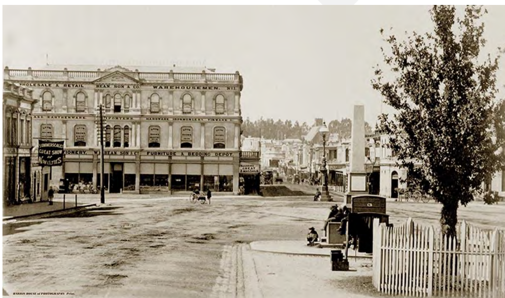
Figure 10. Looking east up Bridge Street, from Sturt Street, 1938. Left is the Victorian building occupied by Bean Son & Co., altered c1960s (as Morsheads Department Store) and c1980s to form Norwich Plaza (Source: Ballarat Revealed).
