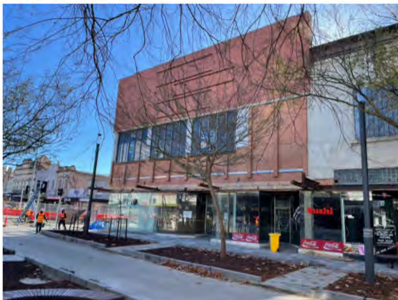
View of the c.1962 building Bridge Mall elevation showing the windows inserted into the façade.
