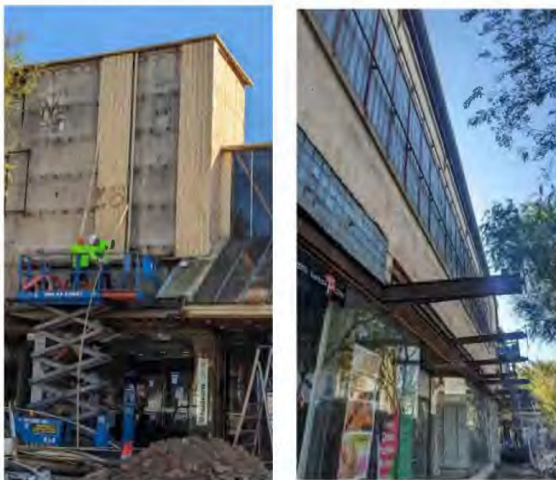
Figure 3 – Existing Eastern portion of Norwich Plaza Southern façade
