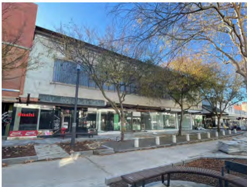
View of the c.1952 building from the south side of Bridge Mall – note section of glass bricks above the shopfronts to the left.
