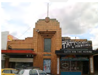
Figure 27. (left) Former North Grant Hotel, 3 Peel Street (GJM Heritage, November 2021).
