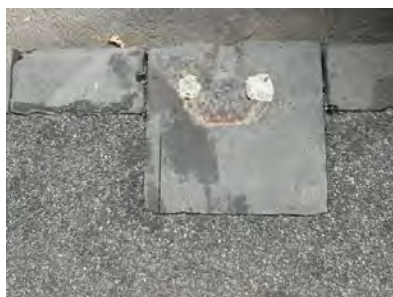
Figure 22. (right) Large kerb block with remnant marks where a verandah post was fixed (City of Ballarat, January 2023).
