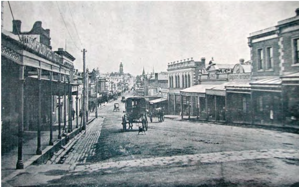
Figure 5. Looking west down Bridge Street from Bakery Hill. On the right are the buildings currently occupied by McDonald's restaurant. Note bluestone kerbs with verandah posts fixed to them and wide bluestone channels along the street [photo undated, prior to Bridge Street tramline installed post-1904] (Source: Victorian Collections, ID 3323).
