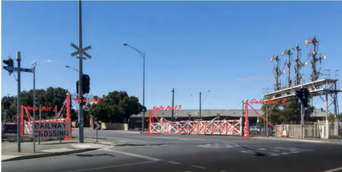
Figure 1. Part of a street view prior to 20 May 2020 looking northeast to the Lydiard Street North Interlocking Sector Gates showing location of gate parts.
