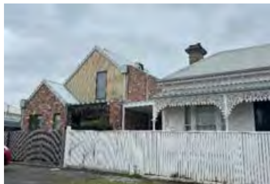
Infill development in Ballarat East
