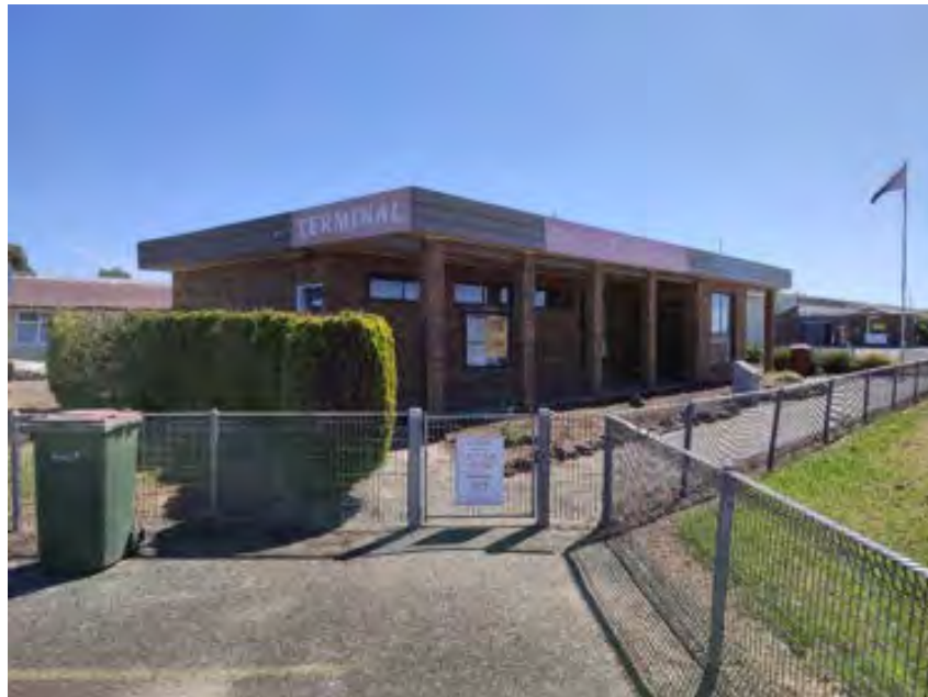
Figure 38: Existing Terminal Building
