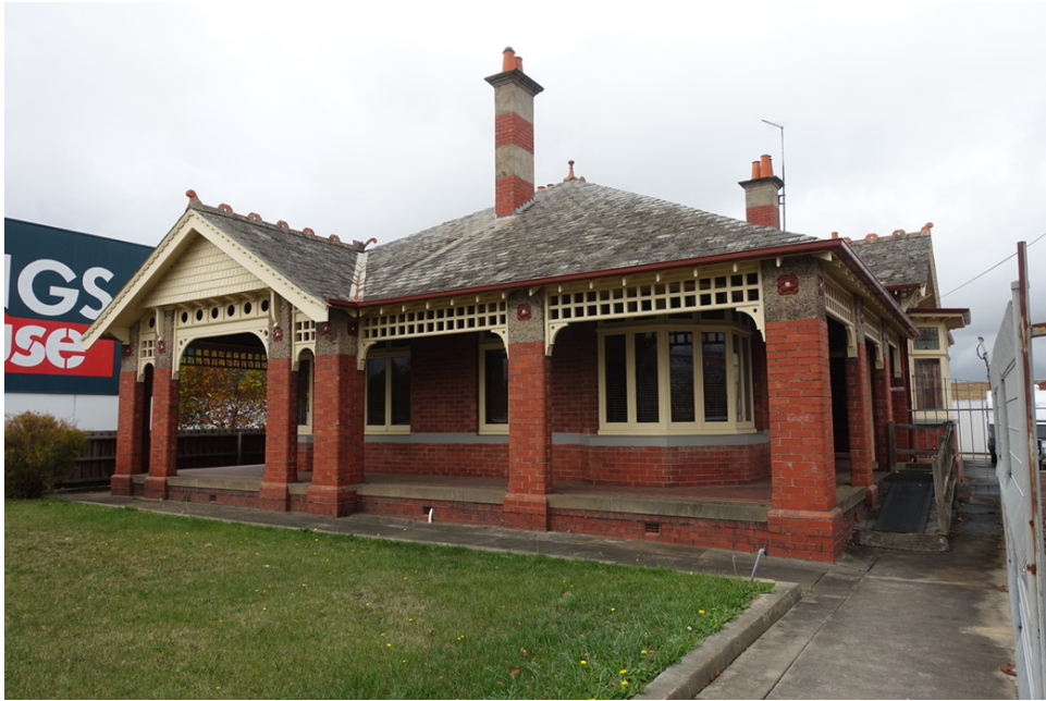
Figure 2 - Front elevation of house at 214 Creswick Road. (Source: Natica Schmeder, 2022)
