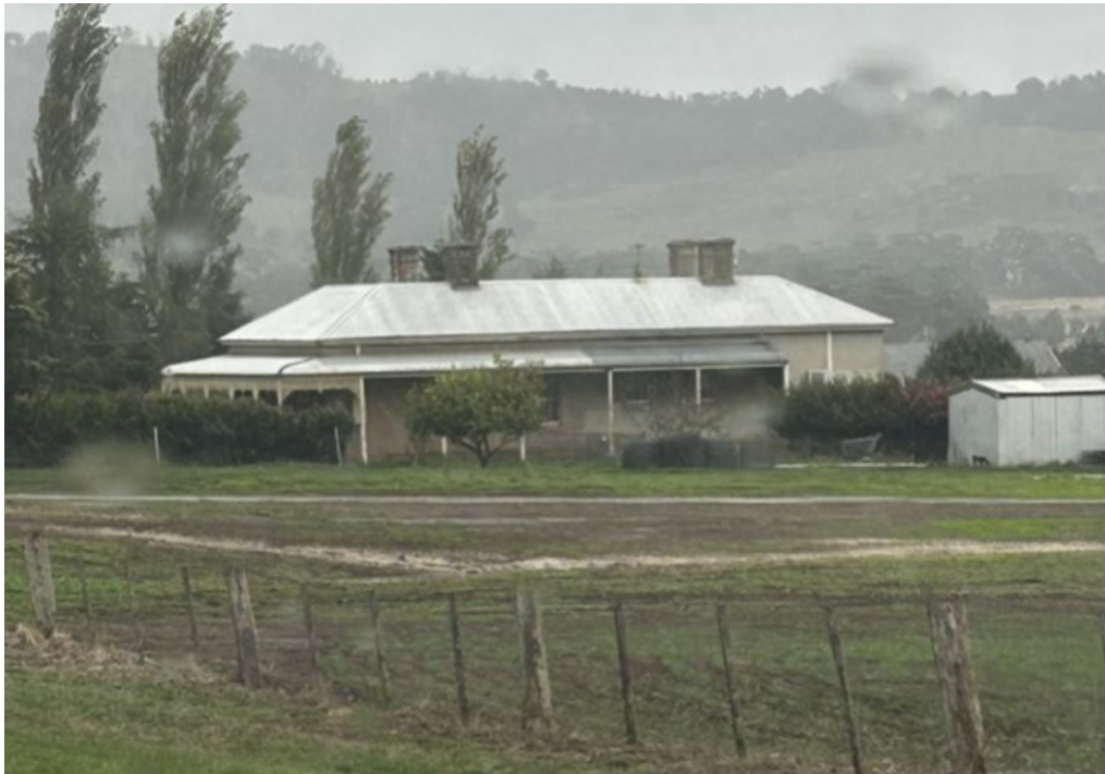
Figure 4 southern elevation of the homestead, showing the two different renders applied to the walls.
