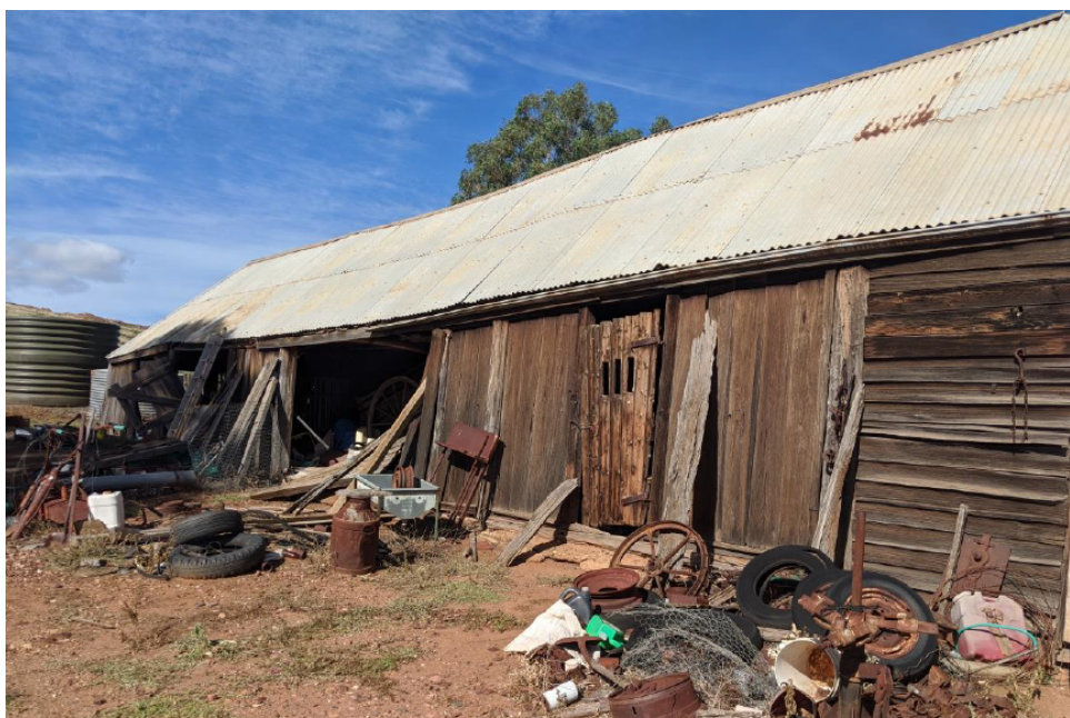
Figure 14 Vallenge's Farm - vertical slab outbuilding
