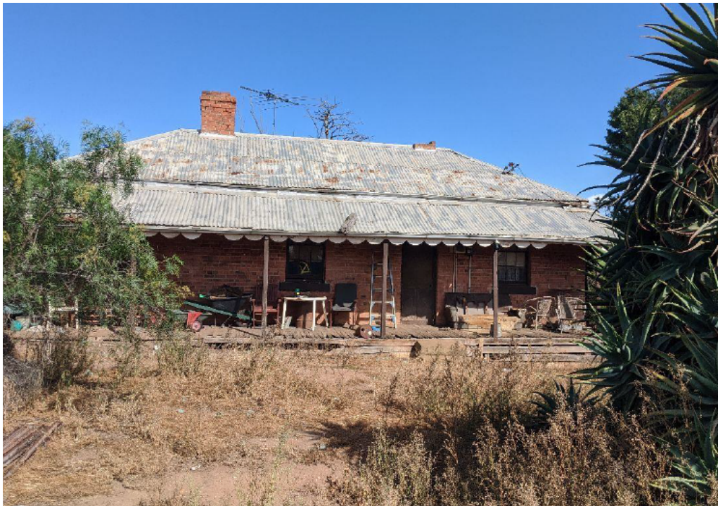
Figure 15 Vallance's Farm Homestead Building (c.1864), included in Moorabool Heritage Overlay (HO174). Source: Heritage Advisor's personal collection, dated 2021.
