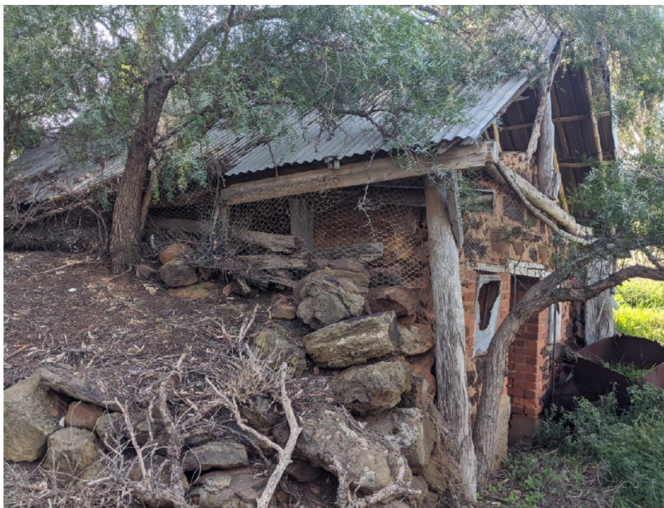
Figure 13 Vallenge's Farm -Subterranean store/dairy . Source: Heritage Advisor's personal collection, 2021.
