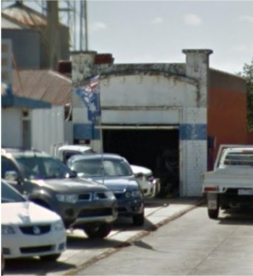
Figure 3 - View of the motor garage from Creswick Road (Source: Google Maps)
