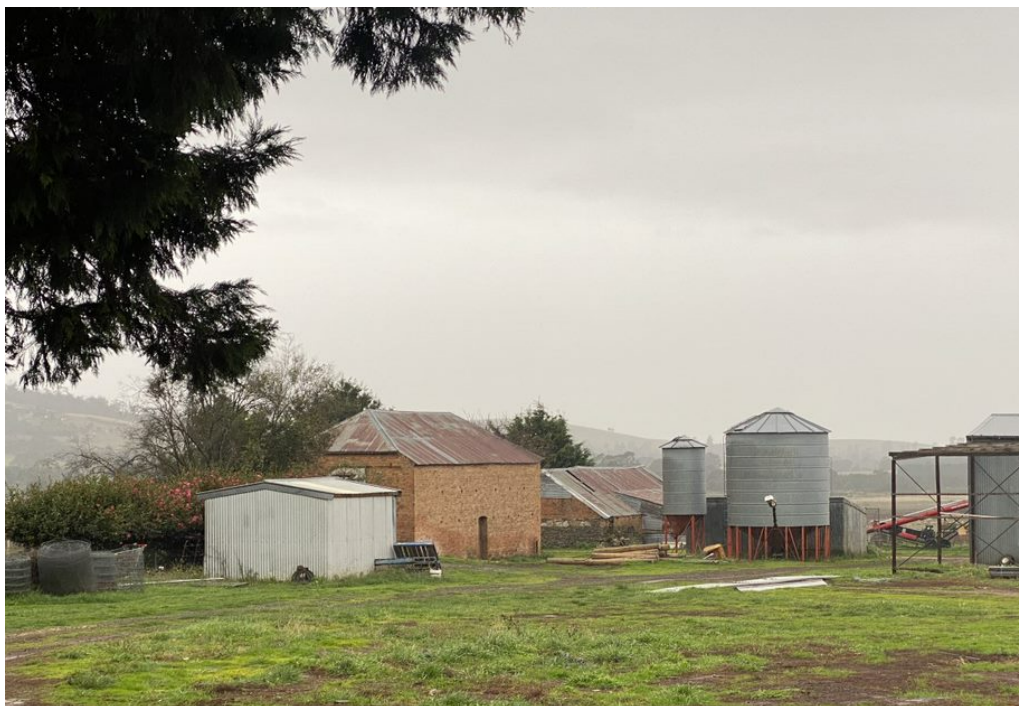
Figure 7 Brick grain store with bluestone and brick outbuilding to the rear.
