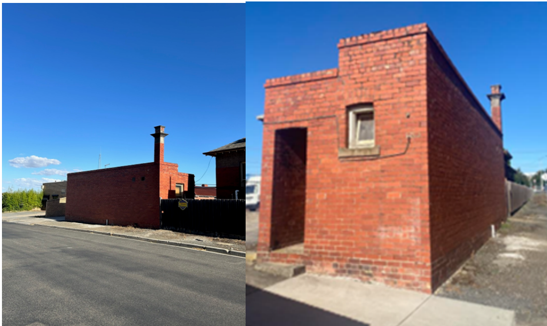
Figure 4 - Images of the laundry outbuilding and a chimney of the dwelling; Source: City of Ballarat, 2024.
