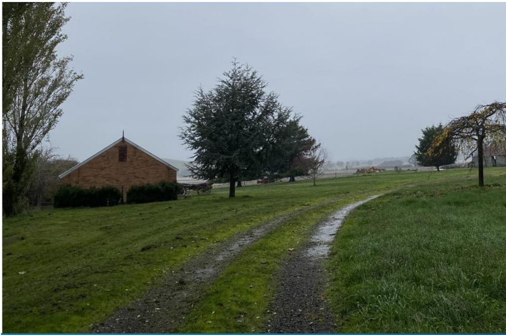
Figure 6 Brick Stable building to the north east of the homestead. Source: City of Ballarat, May 2023
