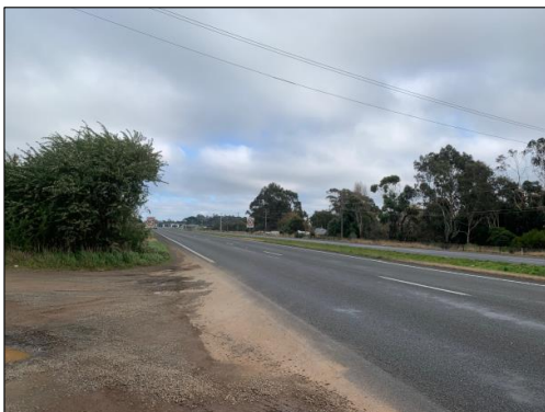
Figure 8: Western Highway (westbound carriageway) - view west
