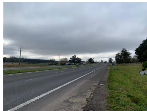
Figure 9: Western Highway (westbound carriageway) - view east
