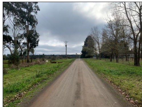
Figure 7: Greene Road - view south
