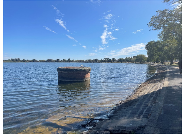
2022, Brick overflow well.
