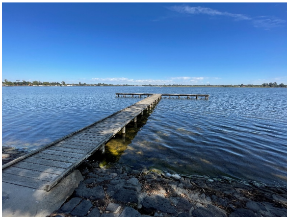
2022, The Ballarat Fly Fishers Club Jetty, erected in 1974.
