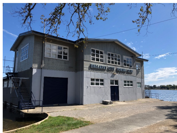
2022, Ballarat City Rowing Club boat shed (rebuilt 1950).
