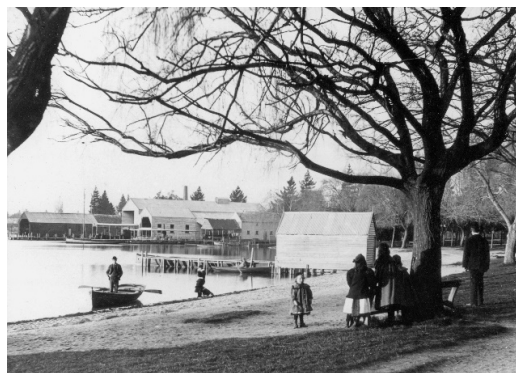
Early twentieth century, Views of the boat sheds.
