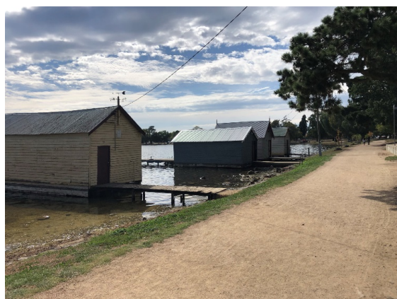
2022, Several of the private boat sheds in the vicinity of the Ballarat Yacht Club.
