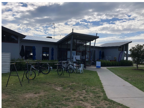
2022, The Ballarat Yacht Club originally constructed 1957-58 and substantially upgraded since 1960s.
