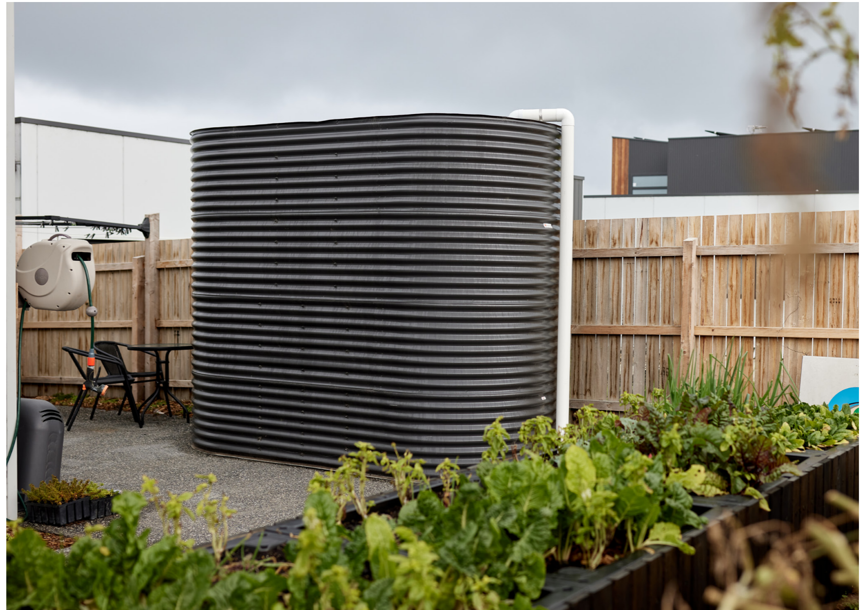
Rainwater tank in rear garden of dwelling at The Cape development. Photography by Kim Landy
