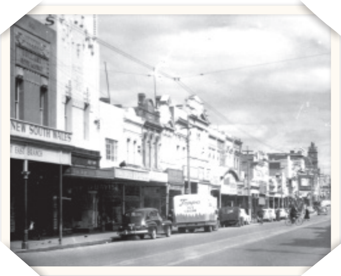
FIGURE 3. Trams, pedestrians and cyclists in former Bridge Street (Bridge Mall) (SOURCES: BRIDGE STREET, BALLARAT, VIC. Rose Stereograph Co c1920-1954. Accession no: H32492/6629. State Library of Victoria)
