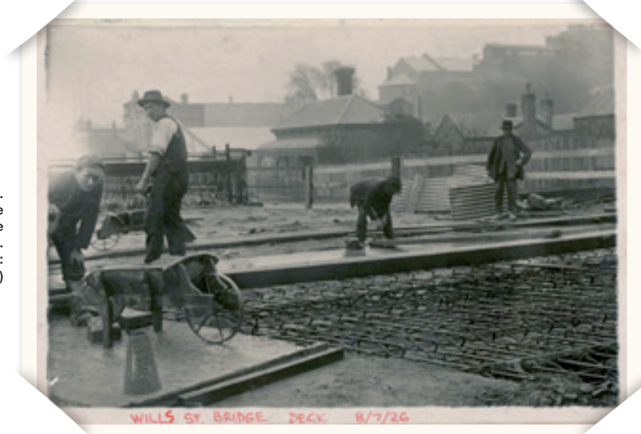
Figure 13. Building the Wills Street bridge deck in 1926. (Image source: City of Ballarat)
