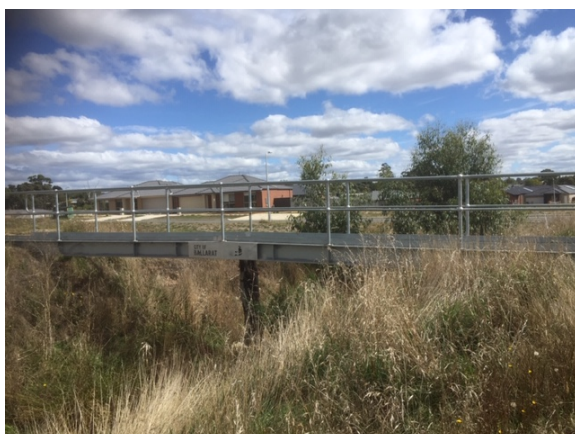
Replacement Bridge at Grasstree Creek
