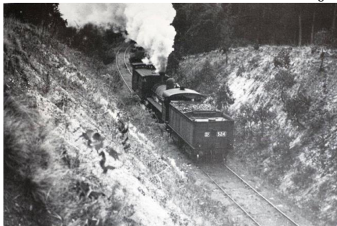
On the bank at Mt Helen, just leaving Buninyong on one of the steepest grades in the district, a 1 in 40. Taken during the War on 13th November 1940.
