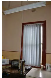
Window detail in office of Administration Building, 2013.
