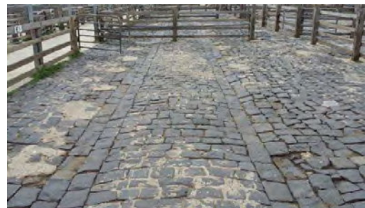
Photo 2: Arrangement of bluestone flooring in the older section of the sheep yard.
