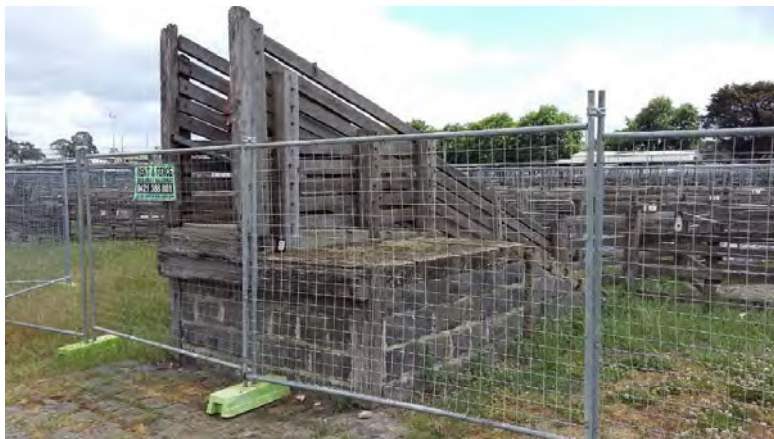
Intact early loading ramp. Note concrete top to original bluestone base, raised to increase height for later stock trucks.
