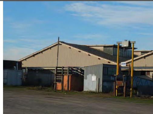
Additional Selling Pavilion, west elevation, 2013.
