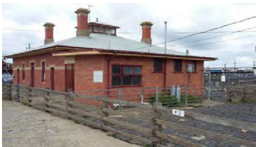
Photo 1: Former Ballarat Saleyards Administrations Building
