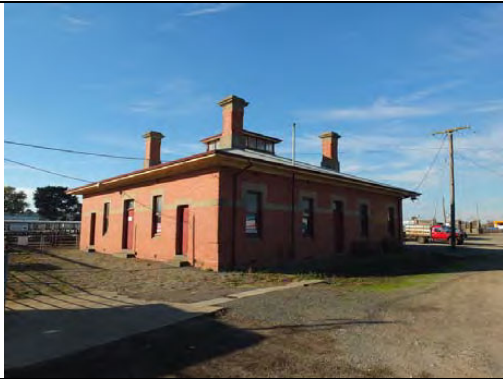
Administration Building, south & west elevations, 2013.
