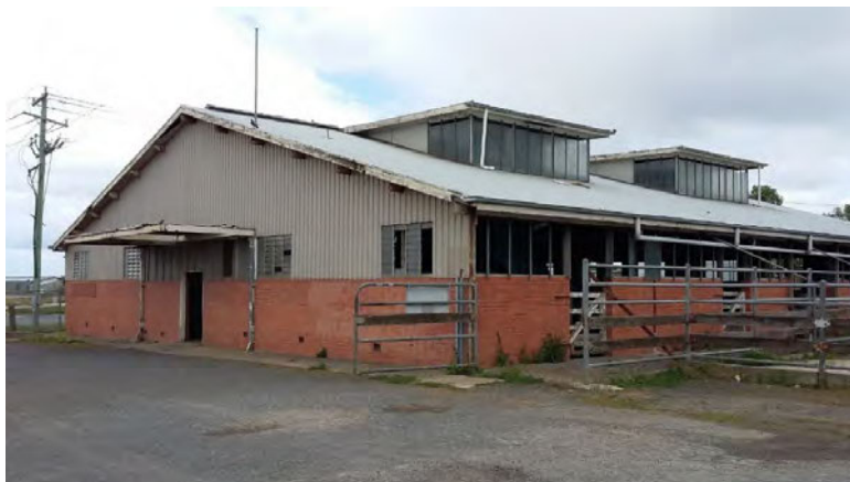
A broad gabled roof form with projecting skillion dormers built c1963.
