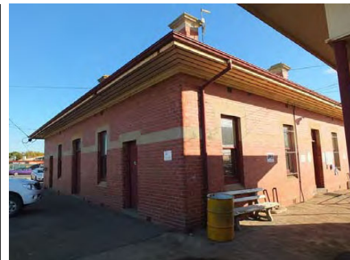
Administration Building, north & east elevations, 2013.
