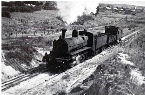
A Ballarat bound ex Buninyong goods in the vicinity of Mt Clear but also looks a bit like terrain between Spencer and Wilson Sts. This picture was taken on the 12th June 1940 by W.Jack.
