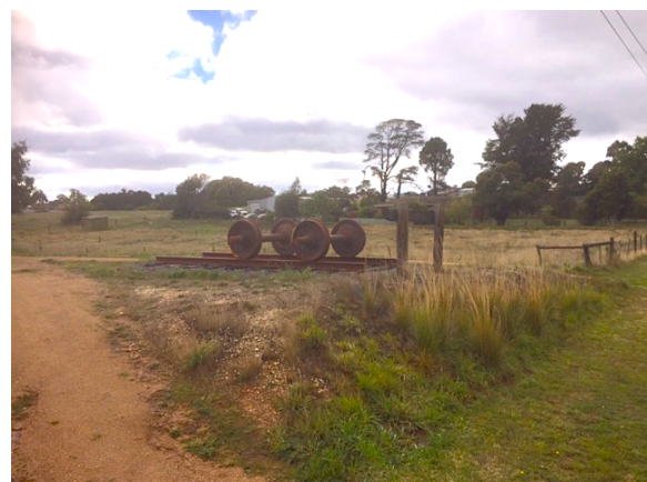
Levy Station and Spencer St bridge abutment.
