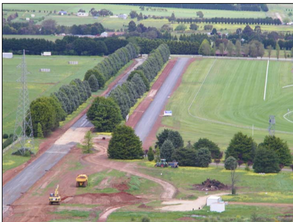
Construction of the new uphill track at Dowling Forest
