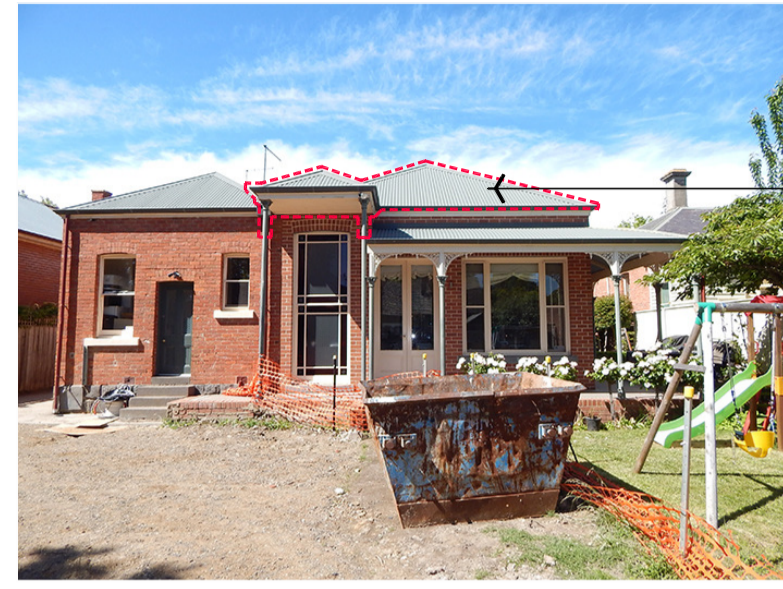
Photo A PROPOSED DEMOLITION
