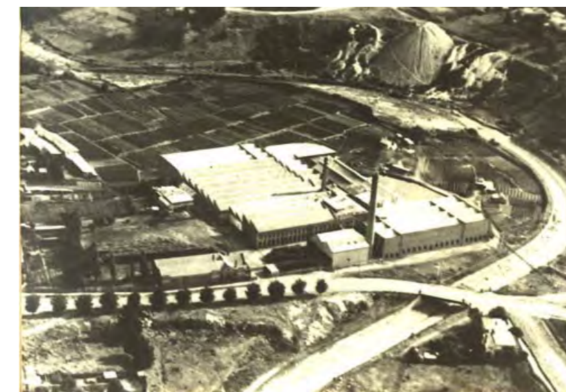
Sunnyside Mill historical photo
