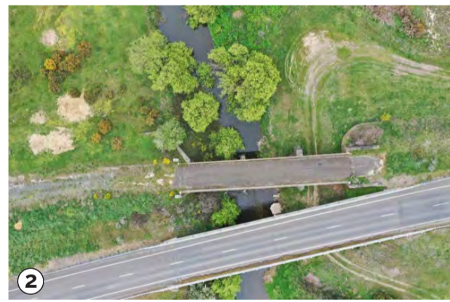
Buninyong - Mount Mercer Road old & new bridges crossing Yarrowee River- edge of COB boundary
