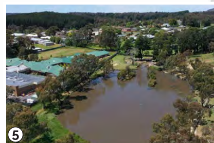
5 Warrenheip Gully dam in Ballarat Wildlife Park
