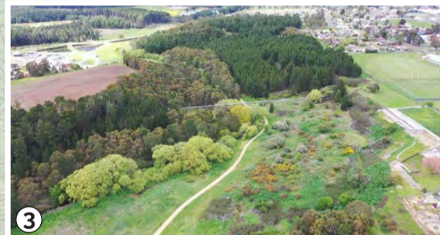
3 Above ground pipe over the river and pine plantation, looking downstream
