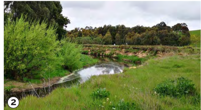
2 Severe erosion along bank
