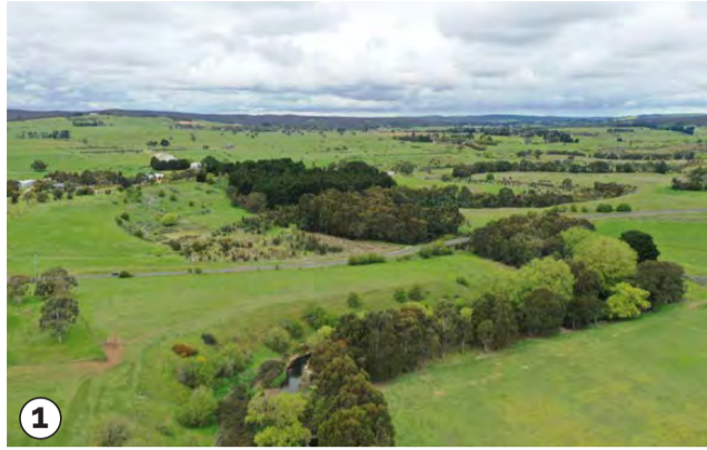
1 Scotchmans Lead Road bridge
