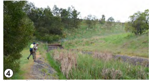
4 Yarrowee River going under freeway
