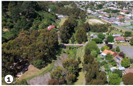
1 Newman Street bridge
