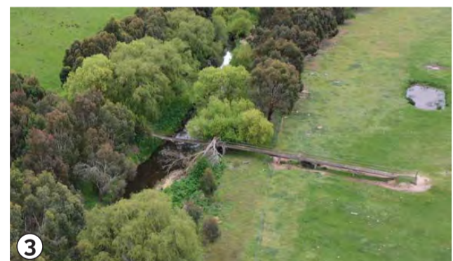
Existing damaged bridge at Glassons Road
