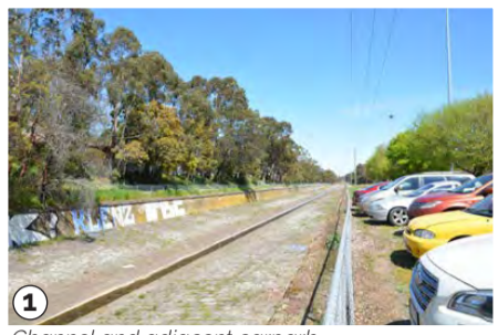
1 Channel and adjacent carpark
