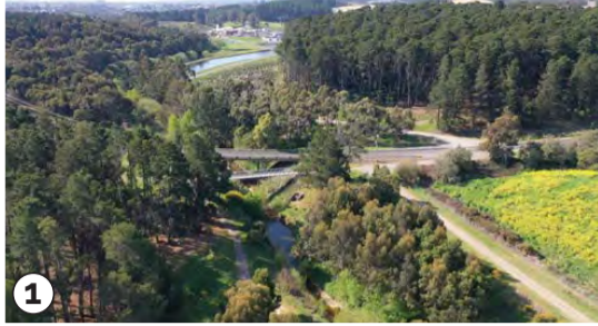
1 Bridge Street / Mount Clear - Sebastopol Road Bridge
