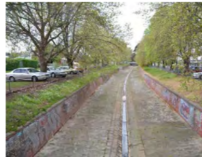
Car parking under large exotic trees in Steinfield Street, Canadian Creek channel.
