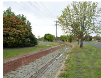
Warrenheip Creek channel on Callow Street
