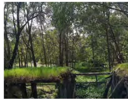
Henderson Lane Bridge and bushland
