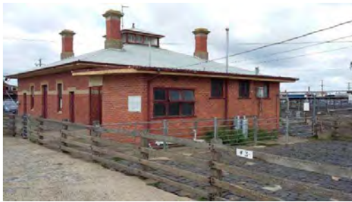
Photo 1: Former Ballarat Saleyards Administrations Building
