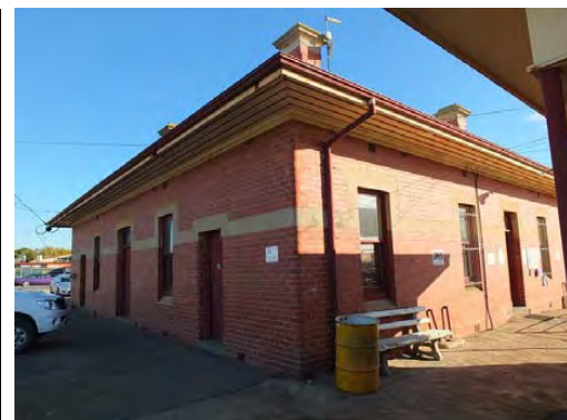
Administration Building, north & east elevations, 2013.
