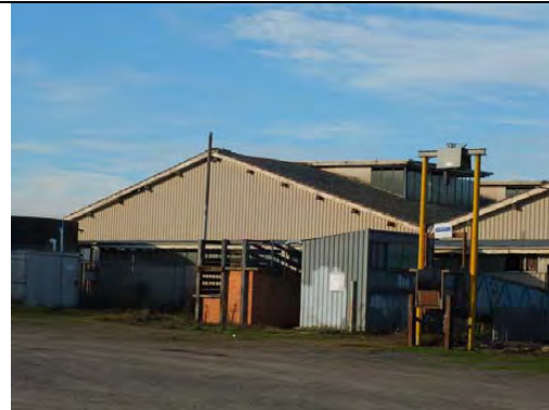
Additional Selling Pavilion, west elevation, 2013.
