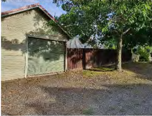
Garage onsite, Eastern Boundary – Facing East
