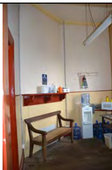
Detail of Blocked up corner fireplace in office of Administration Building, 2013.
