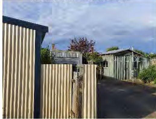
Rear aspect- Southern Boundary
