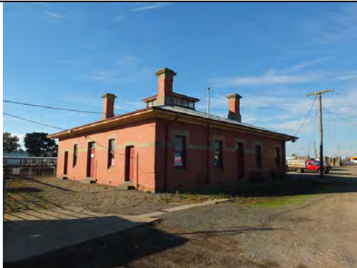
Administration Building, south & west elevations, 2013.
