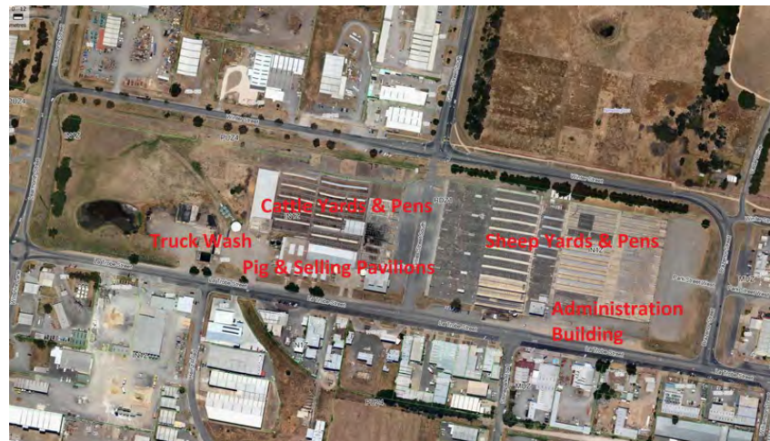
Aerial image of Sale Yards showing the locations of yards and buildings.
