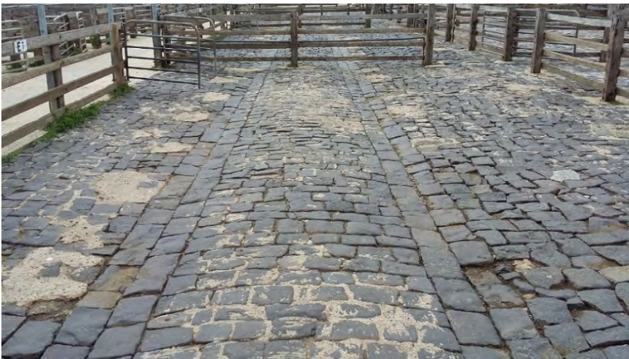
Figure 4: Arrangement of bluestone flooring in the older section of the sheep yard.
