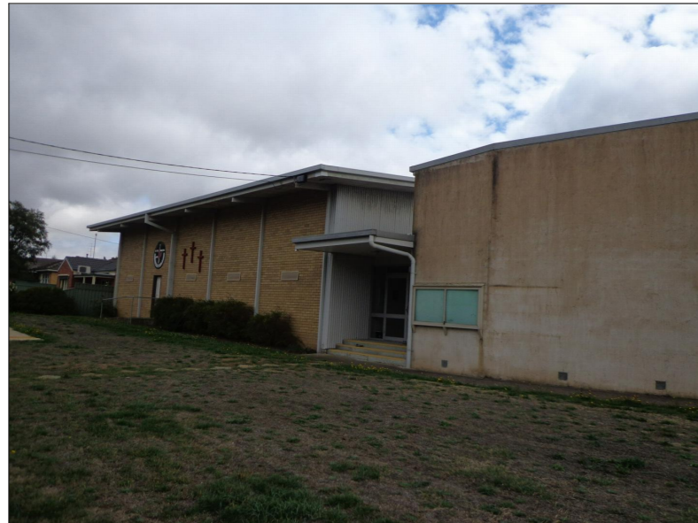
South elevation - Grevillea Road. Fins to be painted colours to match windows. Door set removed and made good with rendered/paint.
