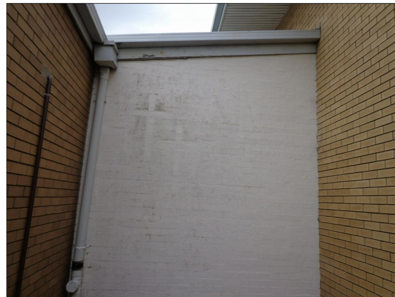
West elevation - Side access door & window to be constructed & rendered & painted grey to match the front of building.
