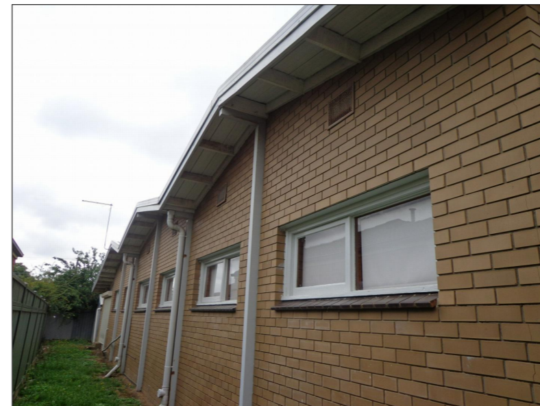
West elevation - No structural change, to be maintained & windows painted where needed.
