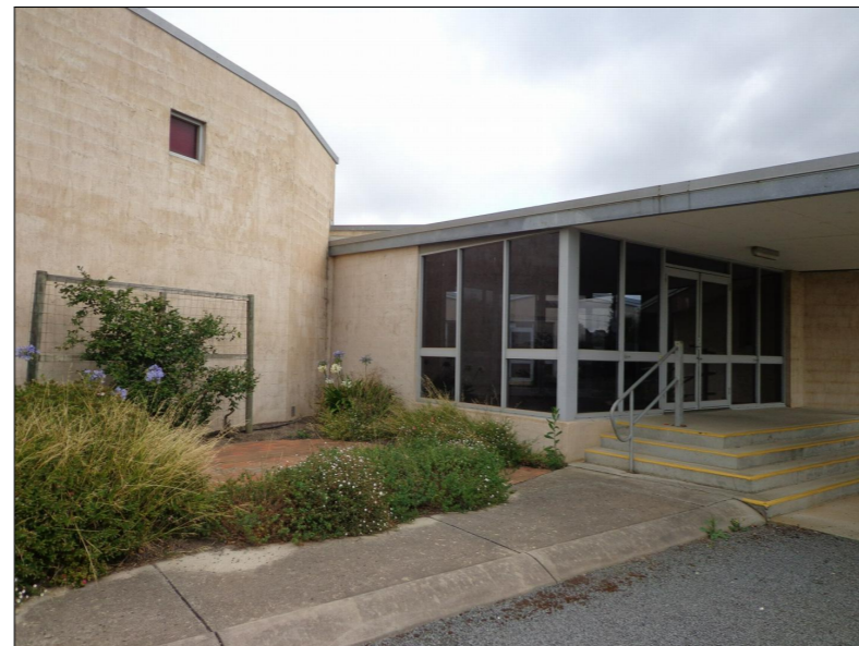
East elevation. Rendered & painted grey, poles painted & 1200h fence added.
