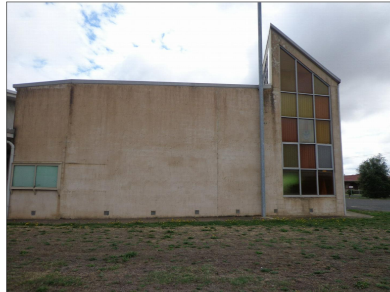
South elevation - Grevillea Road. Render & paint grey. Door/Window combination added.
