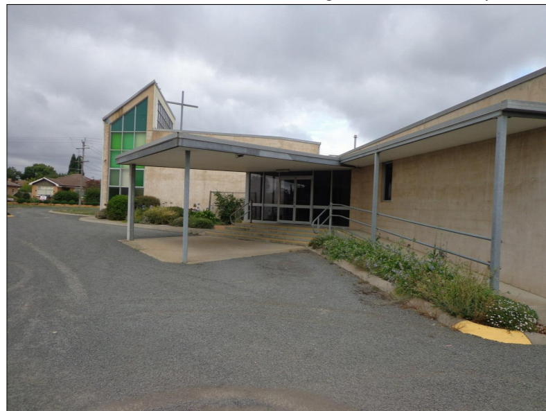
North elevation. Rendered & painted grey, poles painted & 1200h fence added.
