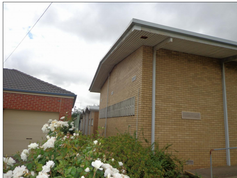
South West elevation - concrete blocks to be removed and replaced with windows & coloured infill panels.
