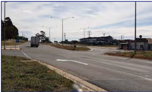
Figure 4: Western Highway view West
