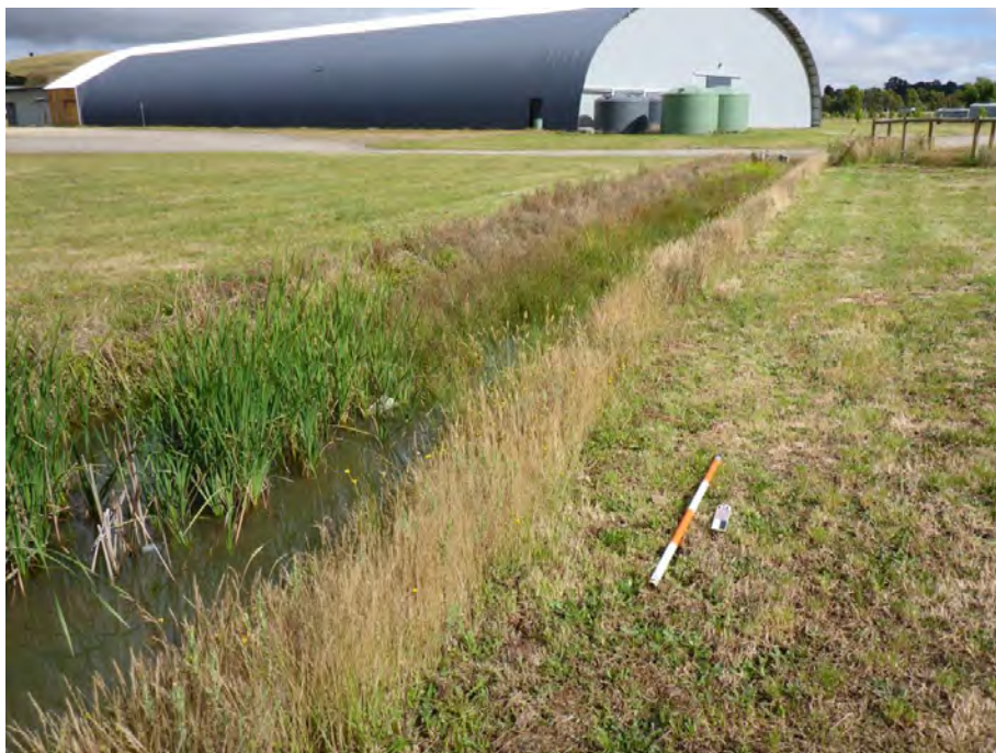
Plate 4: View north along open drain
