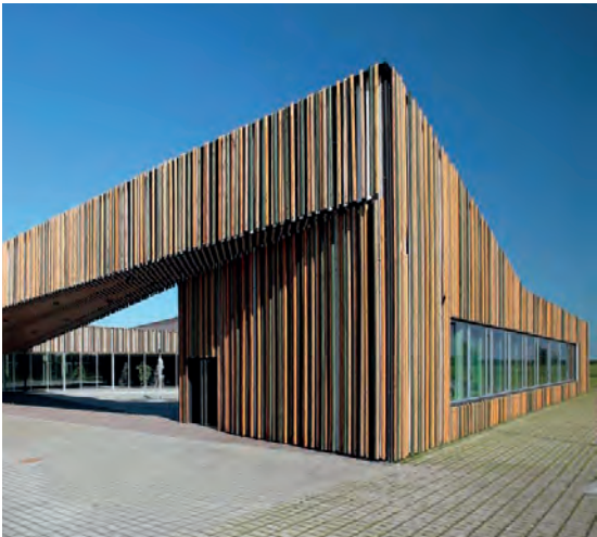
Reference image: potential community facility (Somerru Community Centre)
