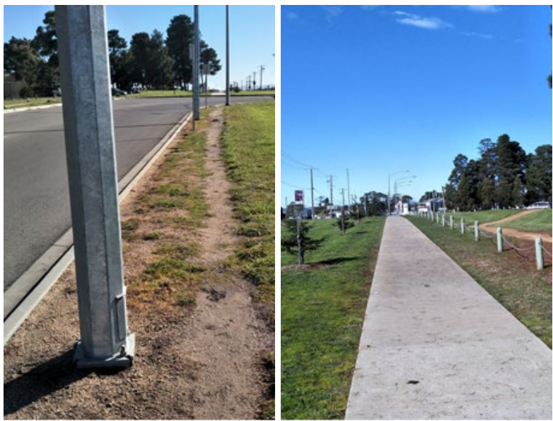
Poor pedestrian infrastructure – lack of pavements, lighting, etc.
