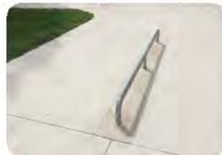
Existing steel rail
