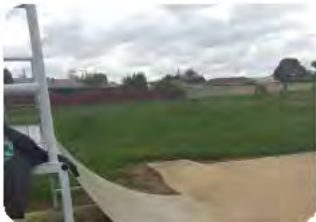
Existing steel ramp
