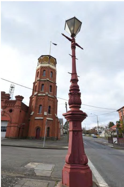
Figure 67: East Ballarat Fire Station
