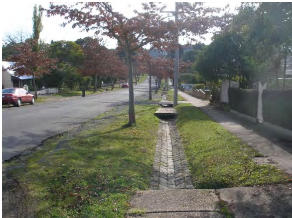
Fig 17: Bluestone channels
