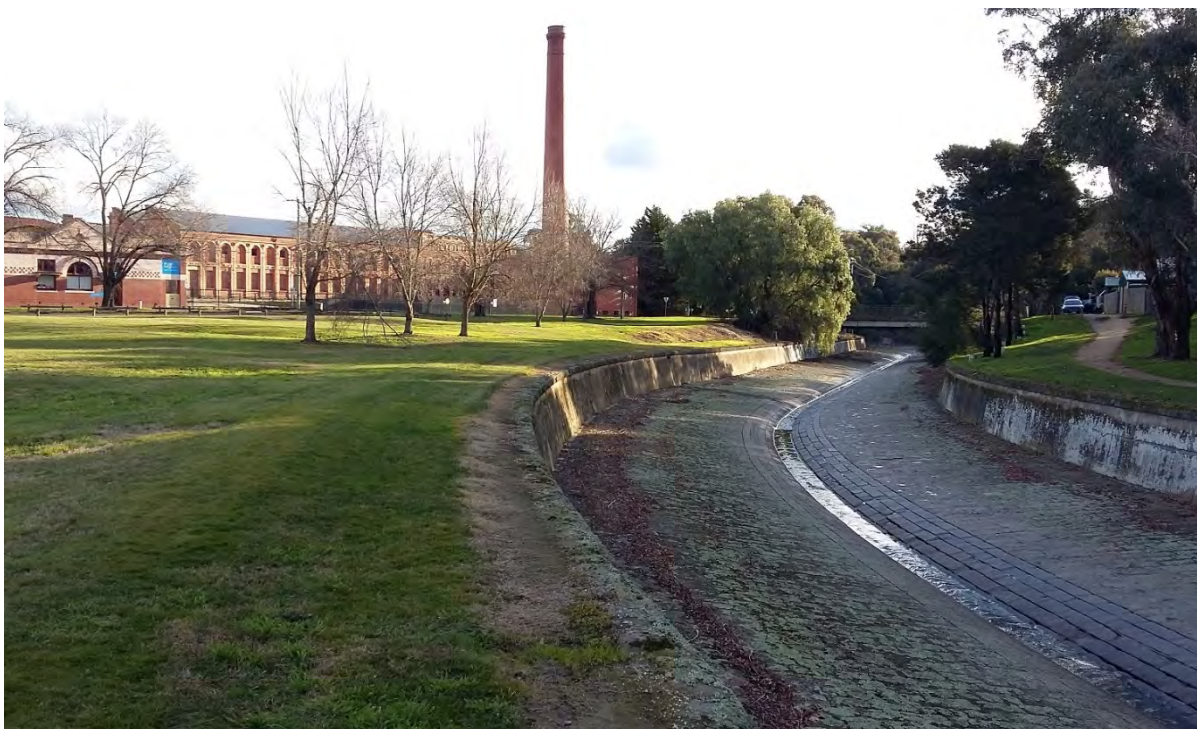
Figure 34: Yarrowee River bluestone channel leading to Sunnyside Mill on Hill Street
