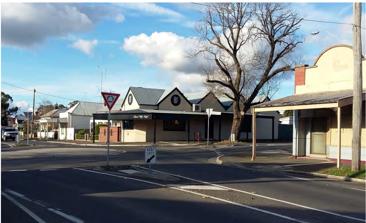
Figure 26: Barkly Street corner shops
