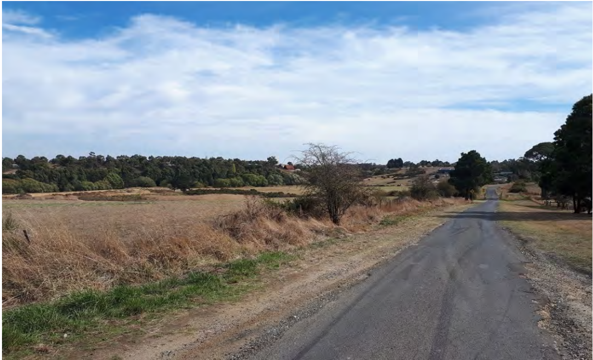
Figure 35: View over the wide river plain to the Redan escarpment from the southern end of Humffray Street South
