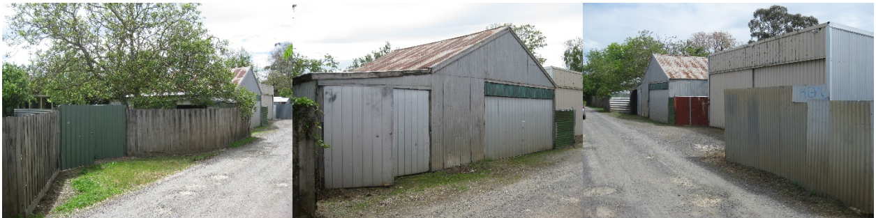
Figure 14: Current southern interface of 1 Murray Street, 17 and 19 Ajax Street with the Right of Way
