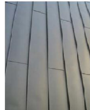
METAL CLADDING TYPE 1 STANDING SEAM COLORBOND FINISH
