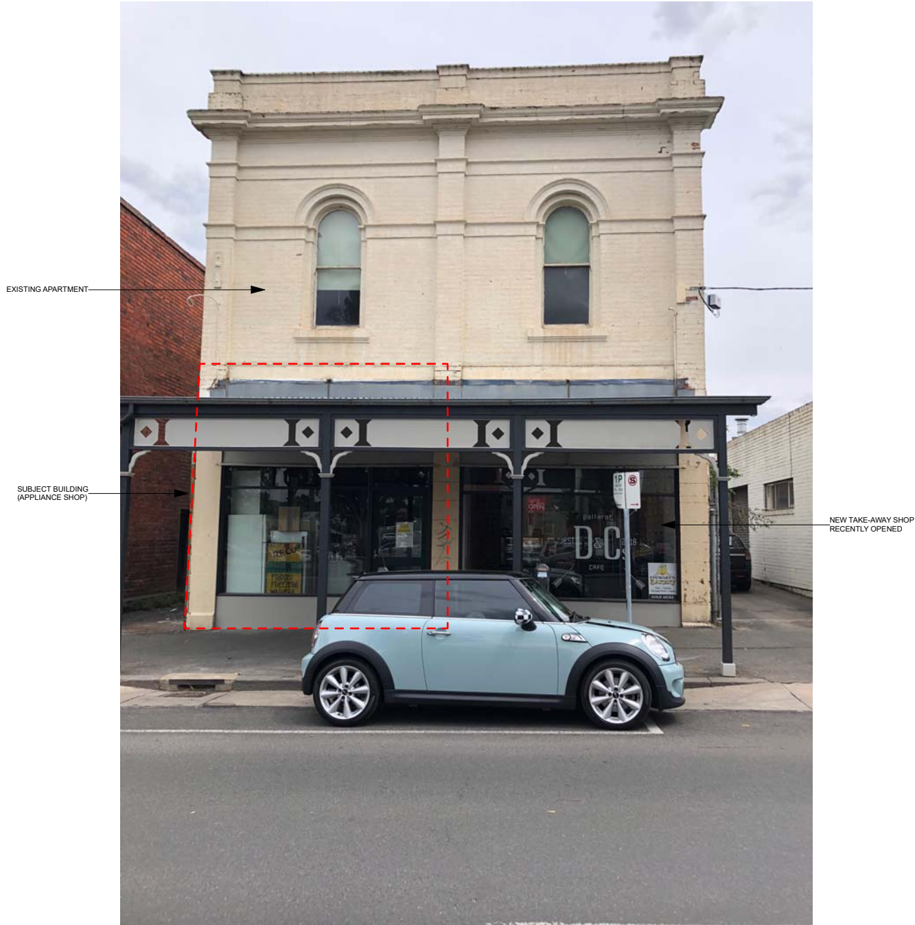
EXISTING FACADE (LOOKING SOUTH)
