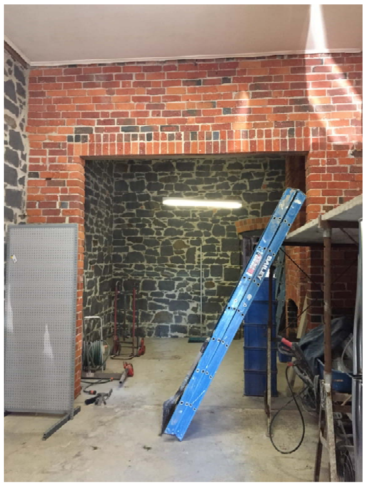
VIEW LOOKING ENTRY DOOR TOWARDS REAR
