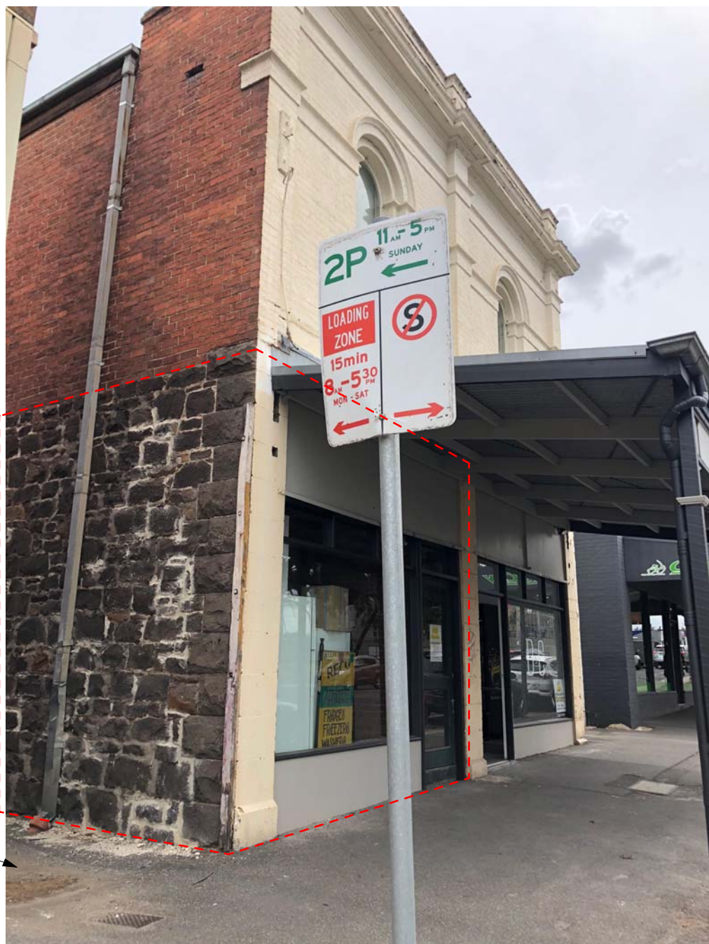
VIEW FROM EAST SIDE OF SHOP LOOKING WEST
