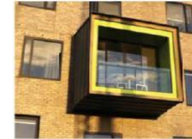
SUGGESTED BALCONY DETAIL & POWDERCOAT ALUMINIUM FRAME WINDOWS
