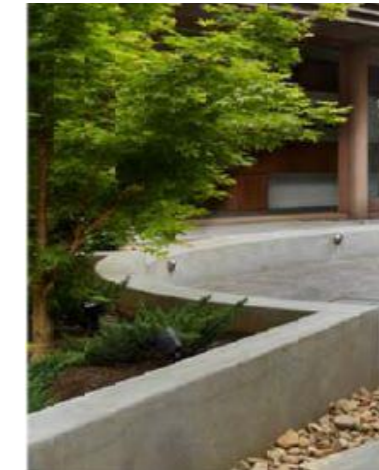
OFF FORM CONCRETE LOW HEIGHT GARDEN WALLS
