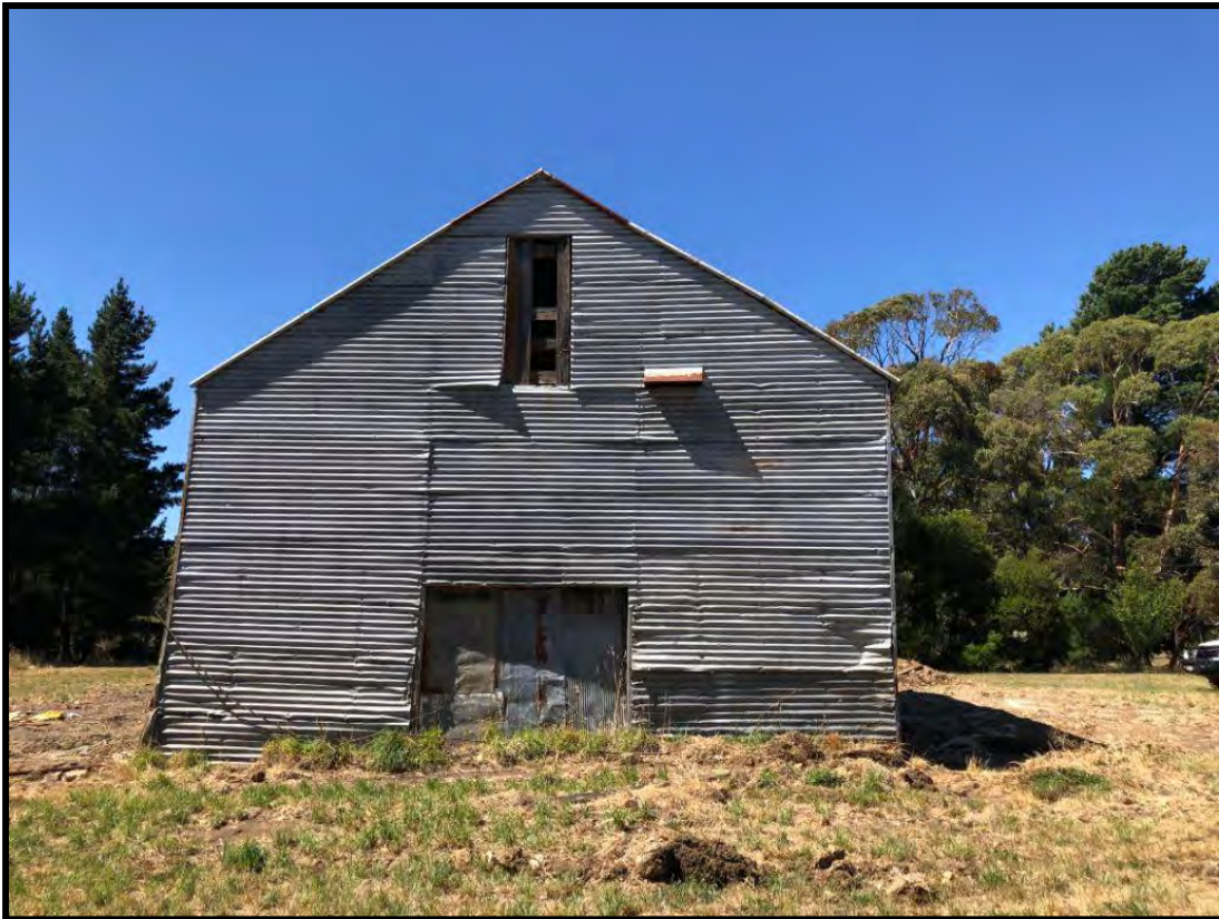
Northern wall, exterior, showing the high window indicative of a winder house (see comparison photos of Wattle Gully Gold Mine, Chewton)
