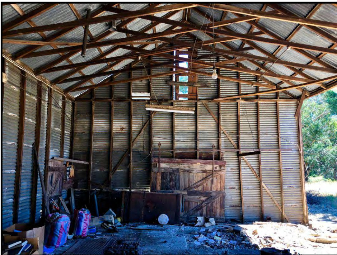
Northern wall, interior, showing haulage window, scissor trusses and wall framing
