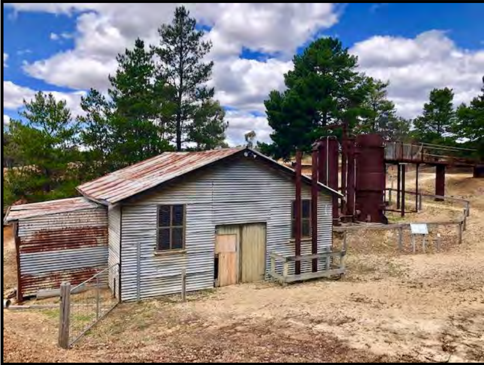
Forest Creek hydraulic sluicing works, Castlemaine – pump shed
