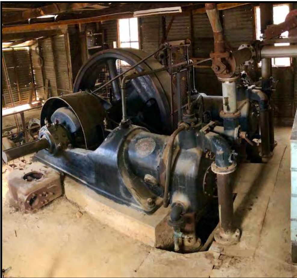
Forest Creek hydraulic sluicing works, Castlemaine – 200hp engine
