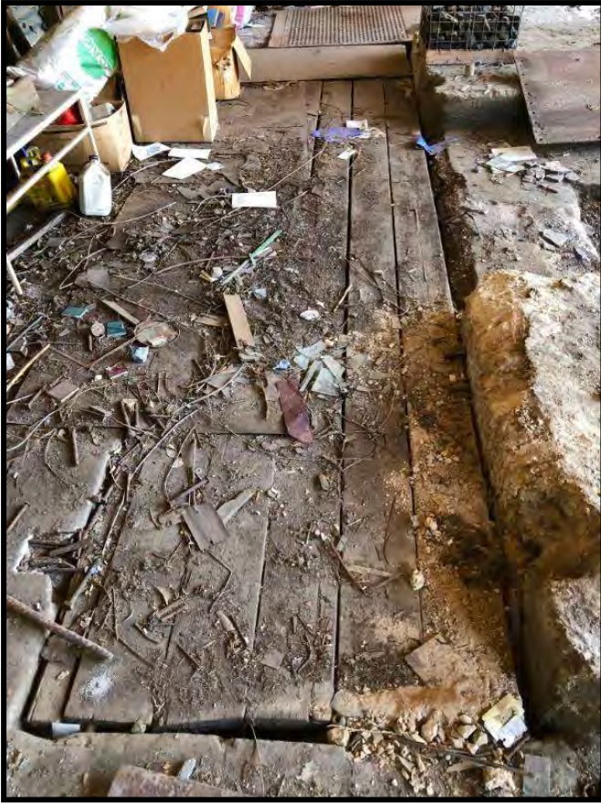
Pit covered by planks and metal grille
