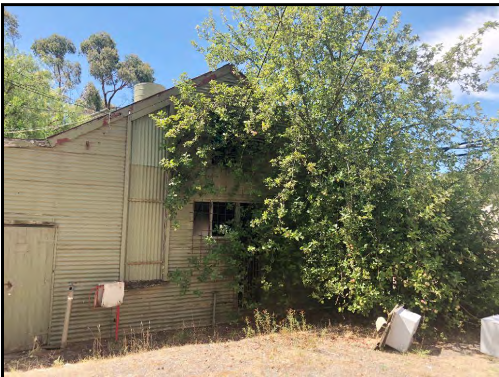
Exterior view of winder house, Wattle Gully Gold Mine
