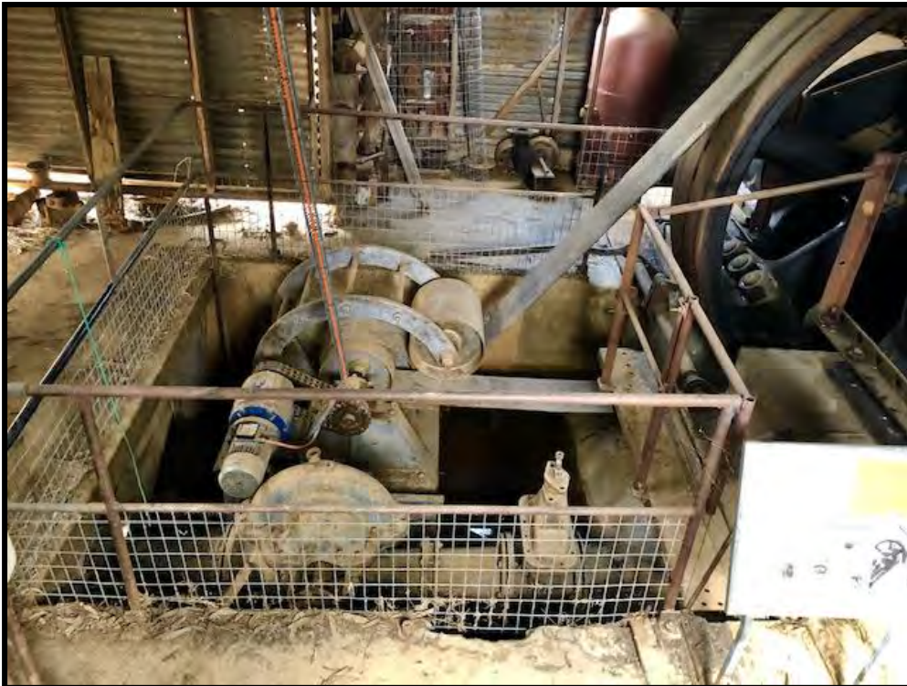
Forest Creek hydraulic sluicing works, Castlemaine – pit at rear of engine for pumping machinery
