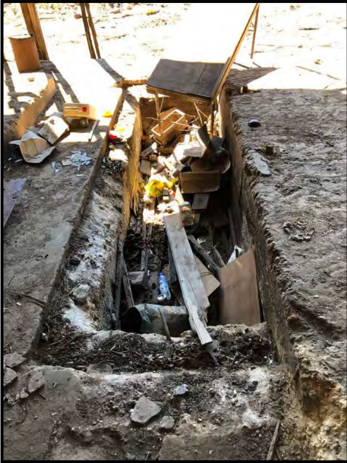
Wheel pit between engine mounting beds
