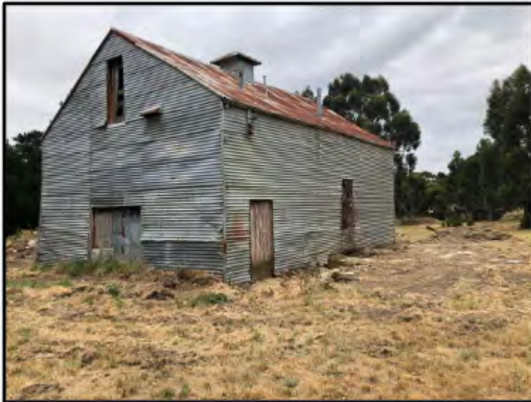
Image: Former Eureka Lead Gold Sluicing Company's pump shed
