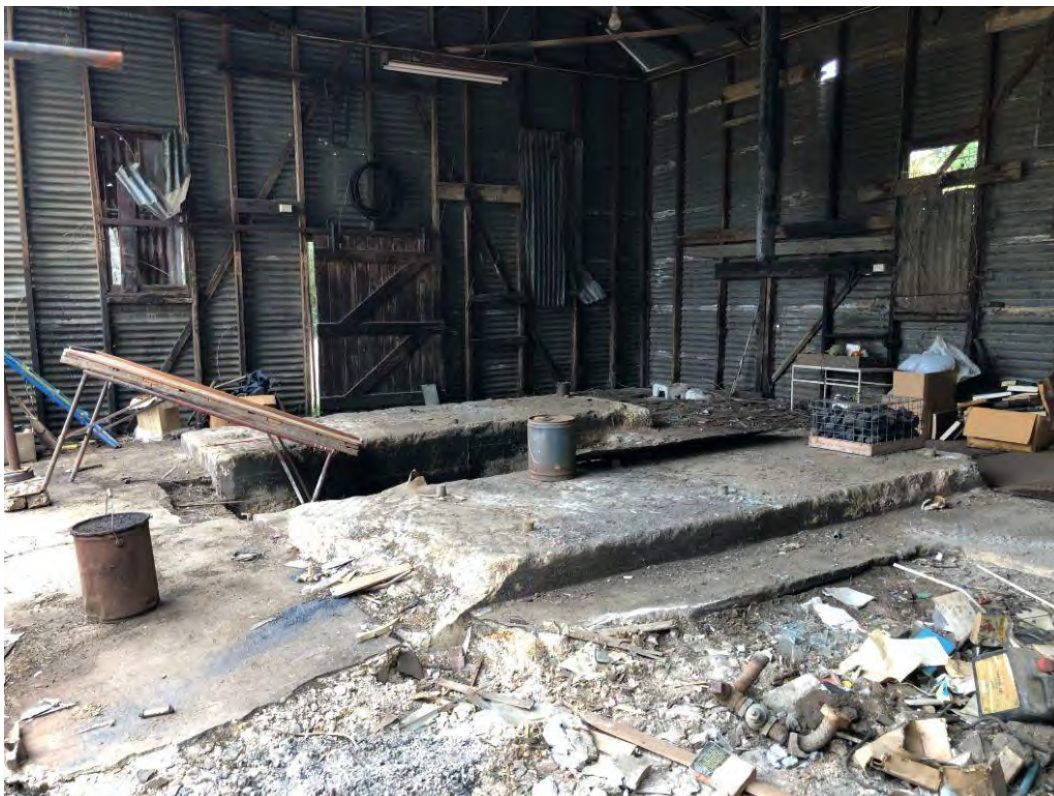
Twin mounting beds for pumping engine
