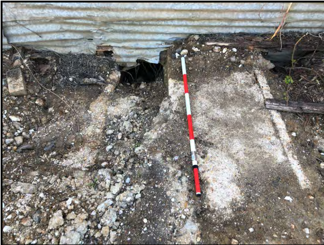
Outline of concrete drain, east side of the shed
