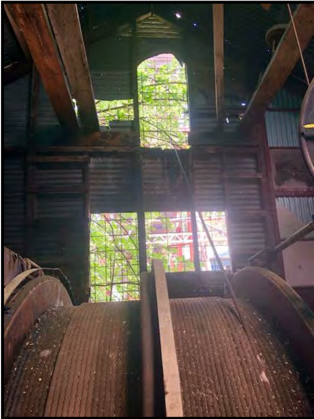
Showing window/entry port for haulage rope, winding engine shed, Wattle Gully Gold Mine, Chewton
