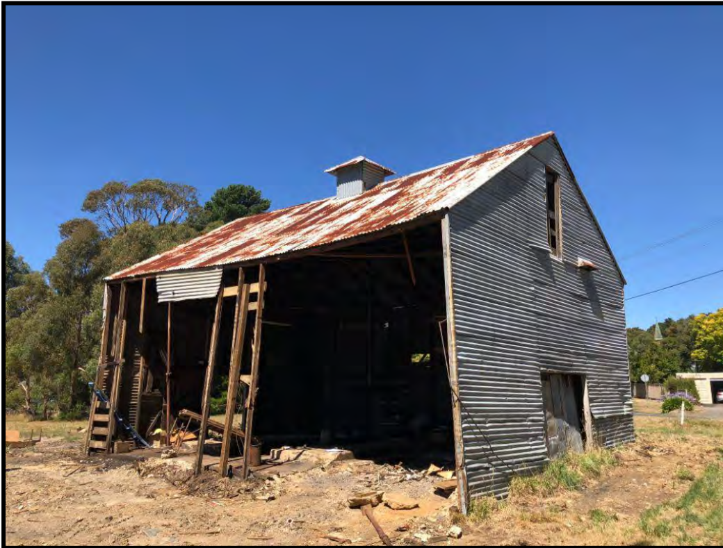
Demolished western wall
