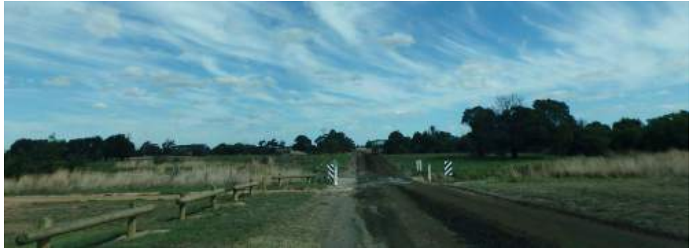
View south along Victoria Street of Burrumbeet Creek road crossing
