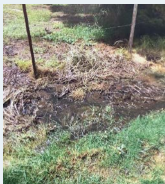
1. Wastewater pooling above ground. (potential for mosquito breeding)
