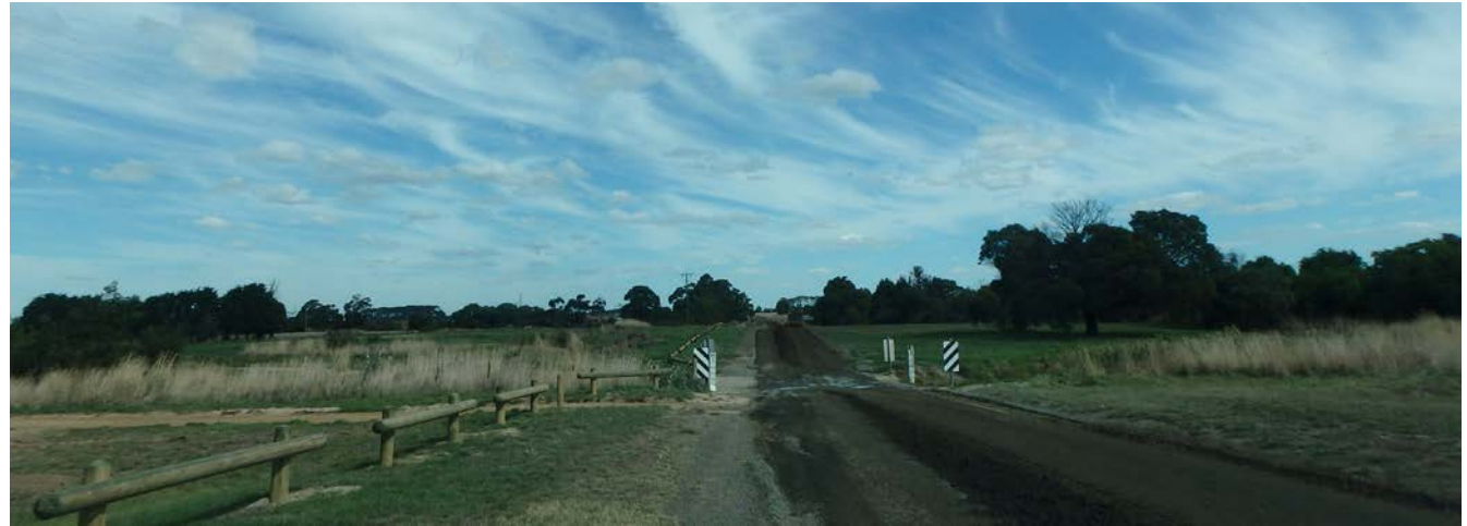
View south along Victoria Street of Burrumbeet Creek road crossing
