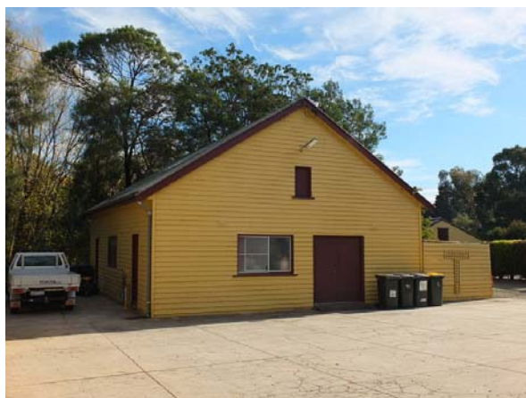
East elevation, Gabled Shed (Building 8).
