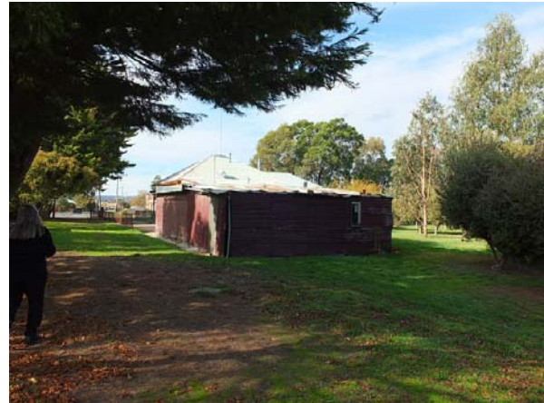
North & west elevations, garage (Building 9).
