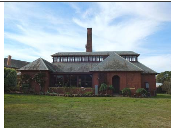
West elevation, former Laundry (Building 7).
