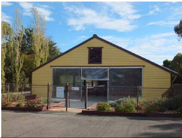
Swimming Pool Enclosure (Building 14).
