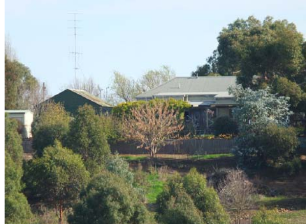
Dwelling, east elevation, 375 Albert Street. (Photograph taken from Magpie).
