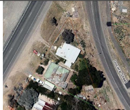
Aerial view of 363 Albert Street. Source: City of Ballarat.
