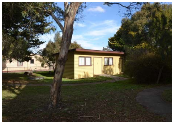
North elevation, former Kindergarten (Building 12).
