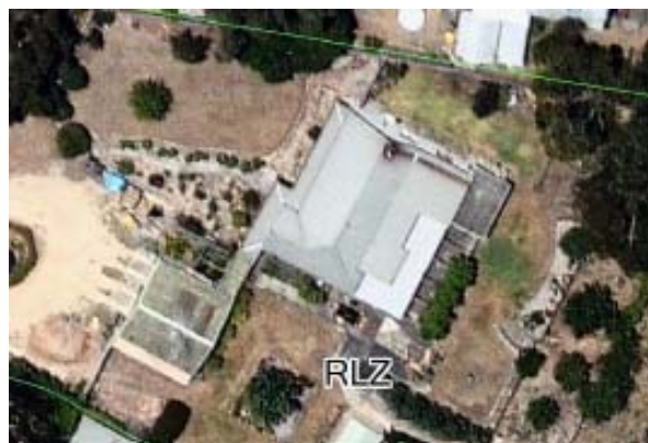
Aerial view of 375 Albert Street. Source: City of Ballarat.
