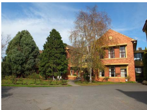
North elevation, Fatima House (Building 10).
