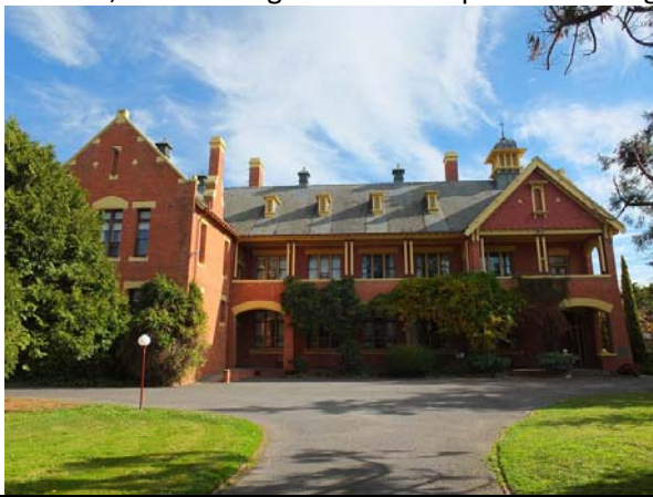
East elevation, St. Joseph's Orphanage (Building 3).
