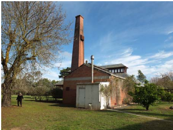
East elevation, Boiler House & Chimney Stack (Building 11).
