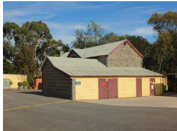
North elevation, Stables & Machinery Shed (Building 2).
