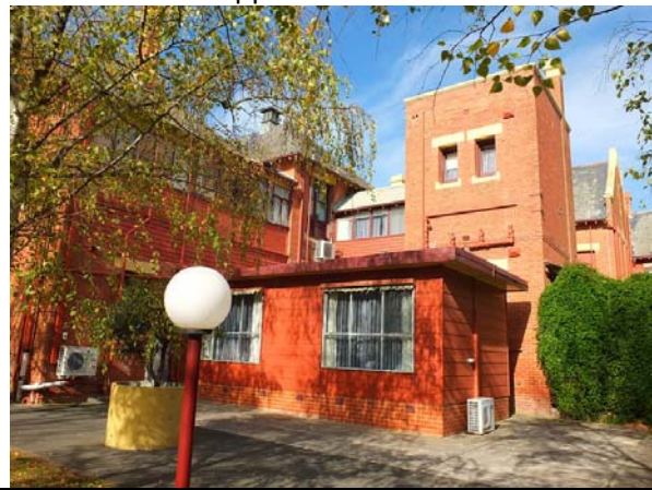
North & west elevations, St. Joseph's Orphanage (Building 3).
