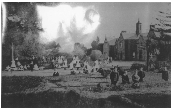
Former Protestant Orphan Asylum & Common School, Fyansford, late 1800s. Source: Geelong Cement Museum.
