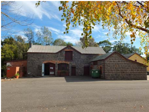
East elevation, Stables & Machinery Shed (Building 2).
