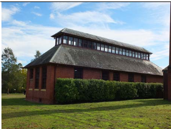
South &amp; east elevations, former Laundry (Building 7).
