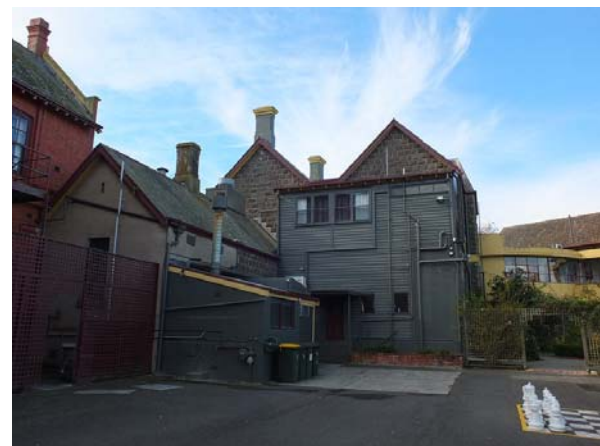
Rear (west) elevation of Blythewood Grange (Building 1).
