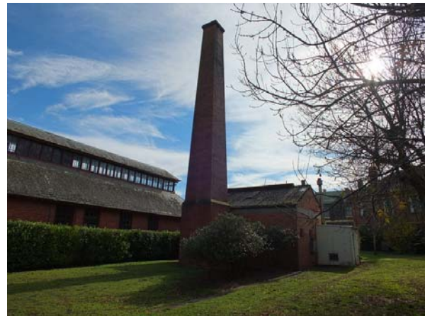
South elevation, Boiler House & Chimney Stack (Building 11).
