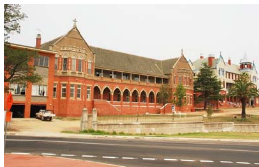
Former St. Aidan's Orphanage, Kennington, 2008. Source: Victorian Heritage Database online.
