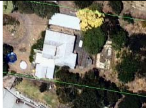
Aerial view of 373 Albert Street. Source: City of Ballarat.
