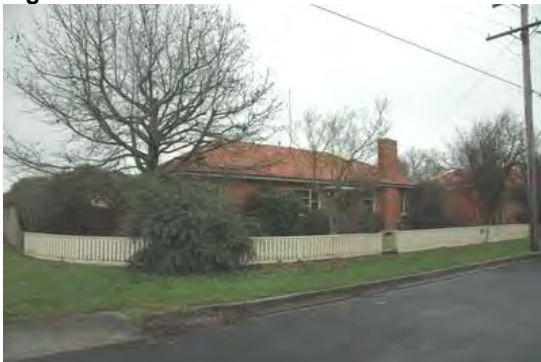
Figure 2.21: Front fence at 10 Exchange Street.
