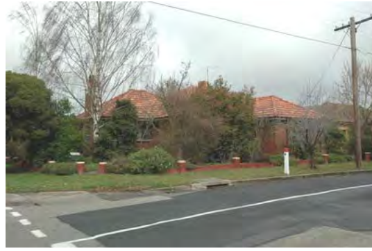
Figure 2.20: Front fence at 8 Exchange Street.
