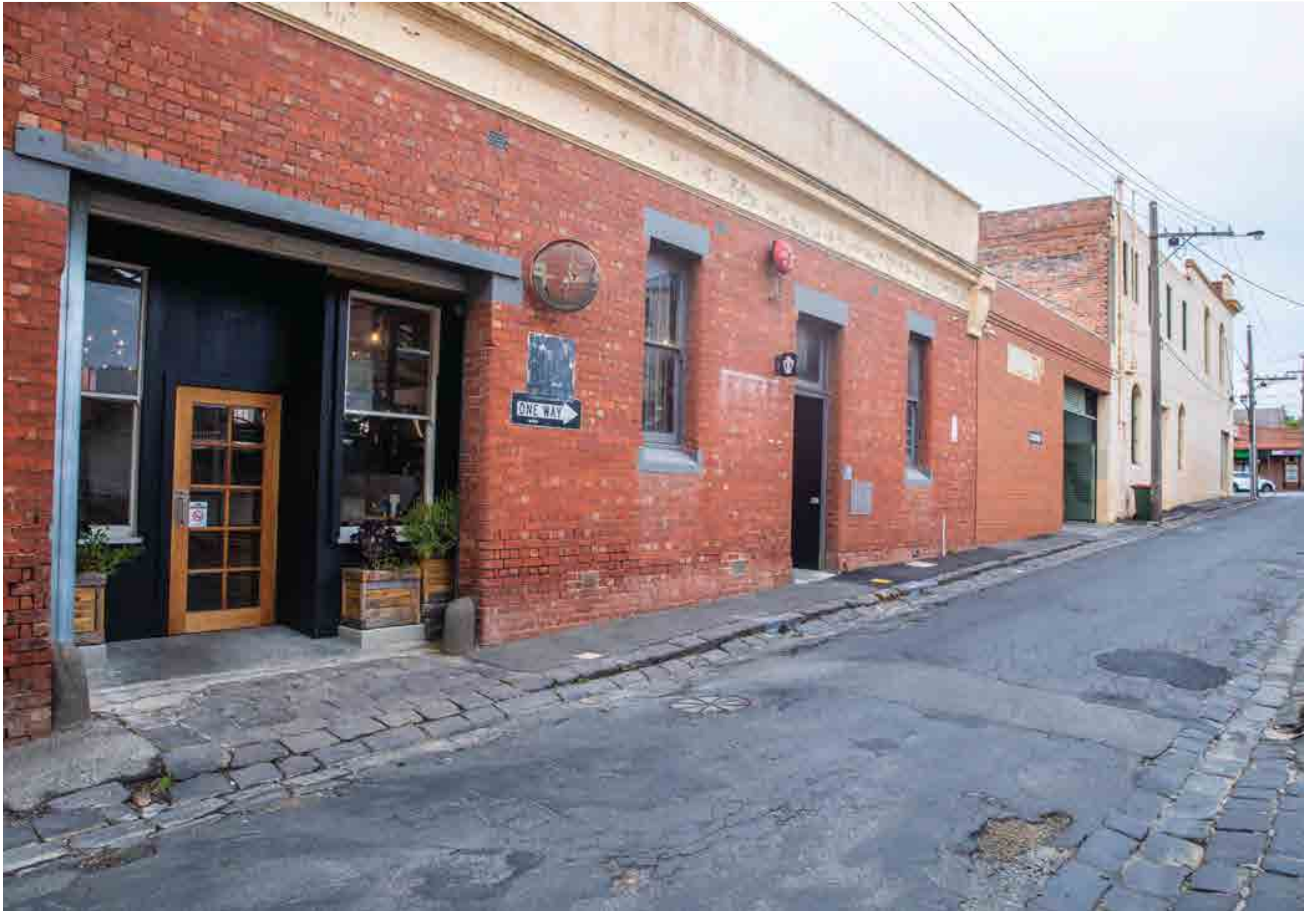
– McKenzie Lane Hydrant Food Hall | Ballarat
