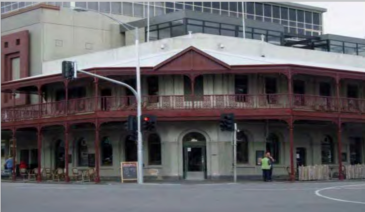
Image: The City of Ballarat's grant program has helped owners undertake large and small-scale conservation works, including reinstatement of this verandah at the former Jackson's Hotel, Lydiard Street, Ballarat.
