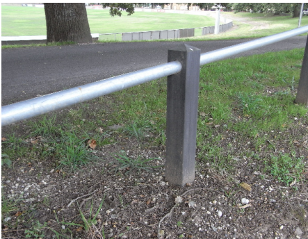
WPC & Galvanised Pipe Fence (Note: photo to be updated) PF 105
