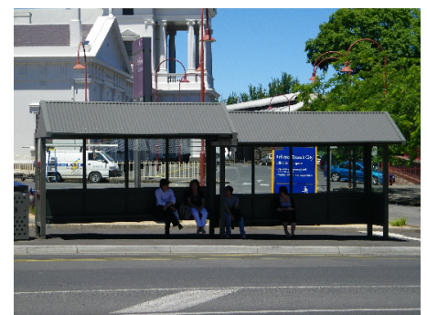
Bus Shelter - Heritage Areas SF 901
