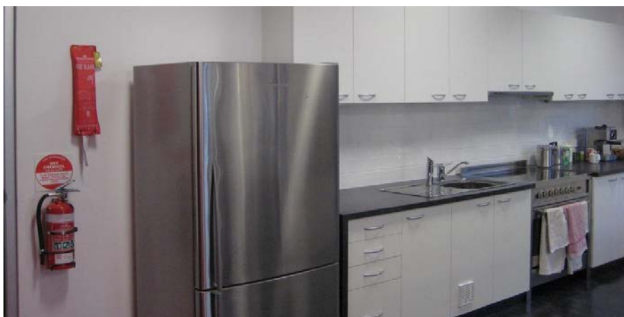
Figure 4: Installation of Fire Extinguisher and Fire Blanket in Kitchen
