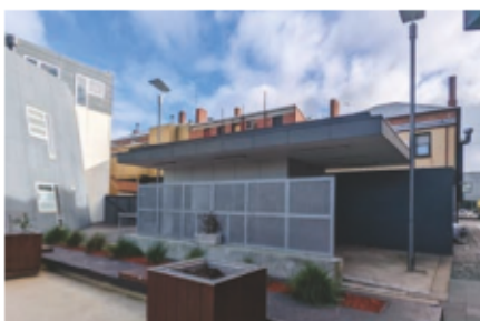
Alfred Deakin Place Public Toilets
