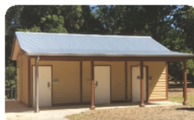
North Garden Accessible Public Toilets
