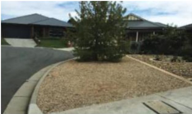
Figure 1 75-100mm of existing turf removed and replaced with compacted aggregate
