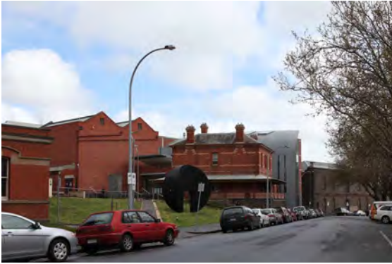
Existing view from the middle of Camp Street looking north-west.
