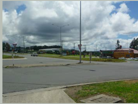
Figure 6 | Intersection of Western Highway & Brewery Tap Road
