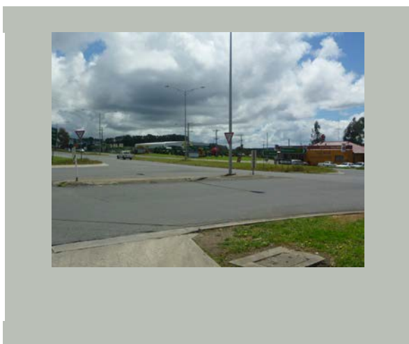
Figure 19 | Intersection of Western Highway and Brewery Tap Road
