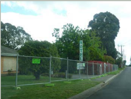
Figure 11 | Redundant motel use
