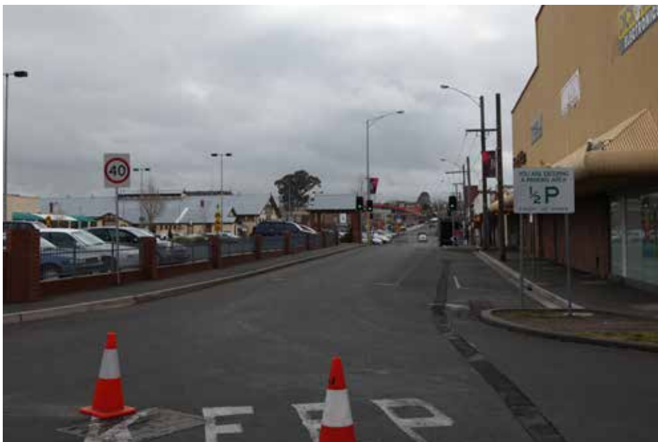
Existing view from Grenville Street looking east along Curtis Street.
