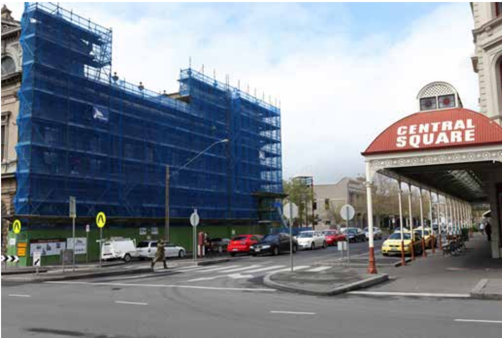
Existing view from Sturt Street looking south along Armstrong Street.
